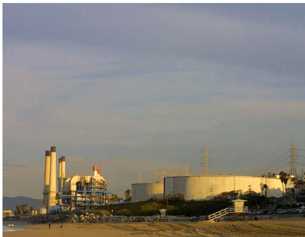
Figure 31. The 113 MW Punta Prieta oil fired powerplant is located on the Baja Peninsula. Note the large oil storage tanks. Image from Photospin.com
