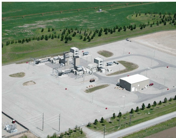
Figure 28. This 2 unit 166 MW natural gas CT powerplant is located near Rathdrum, Idaho. Photo courtesy of Avista Corporation.
