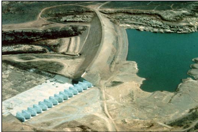
Figure 1.6.1-6. Labyrinth crest (uncontrolled) spillway, Ute Dam, New Mexico.
