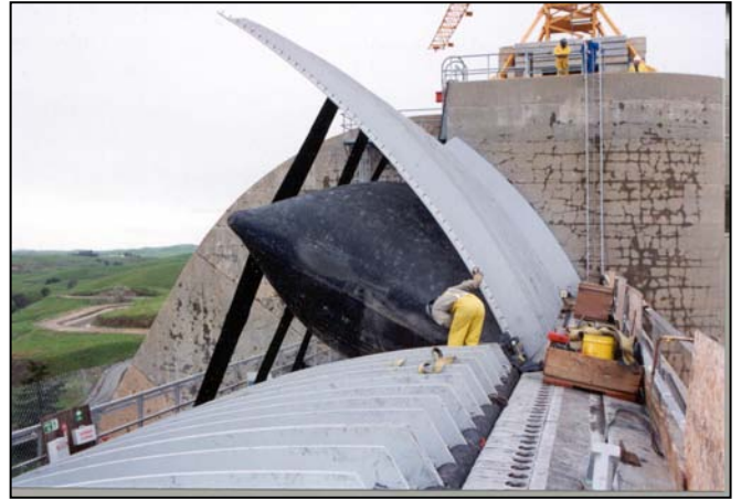
Figure 1.6.1-8. Crest (Obermeyer type) gated (controlled) spillway, Friant Dam, California.
