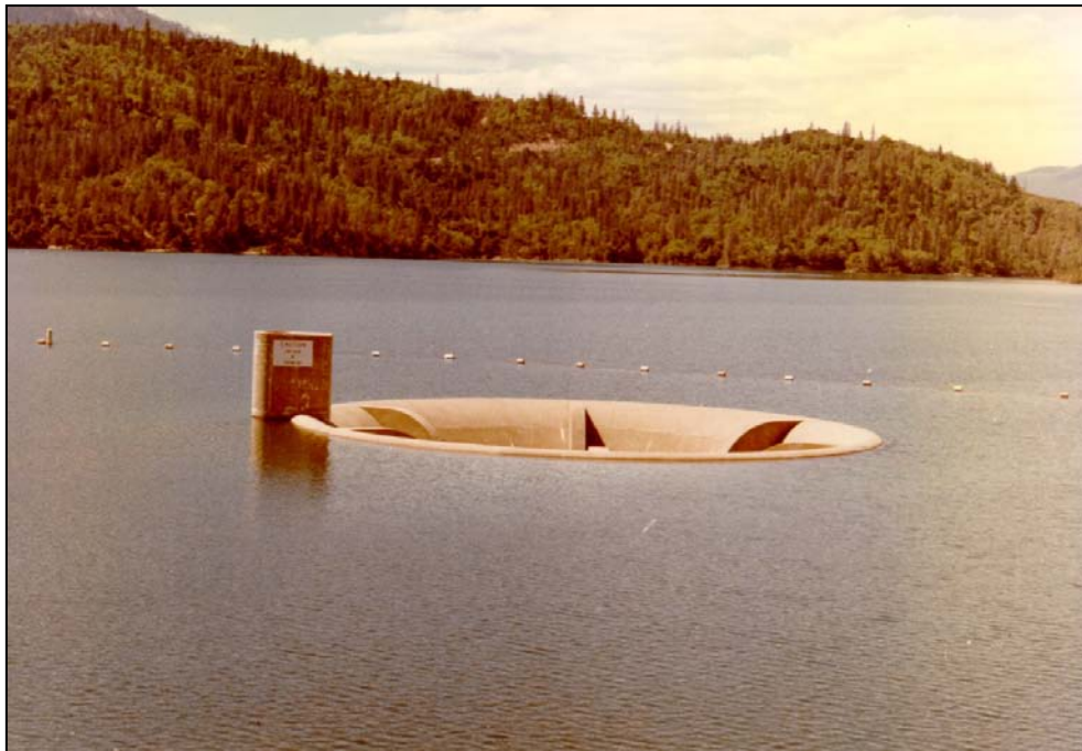
Figure 1.6.1-5. Morning glory (glory hole) crest (uncontrolled) spillway, Whiskeytown Dam, California.
