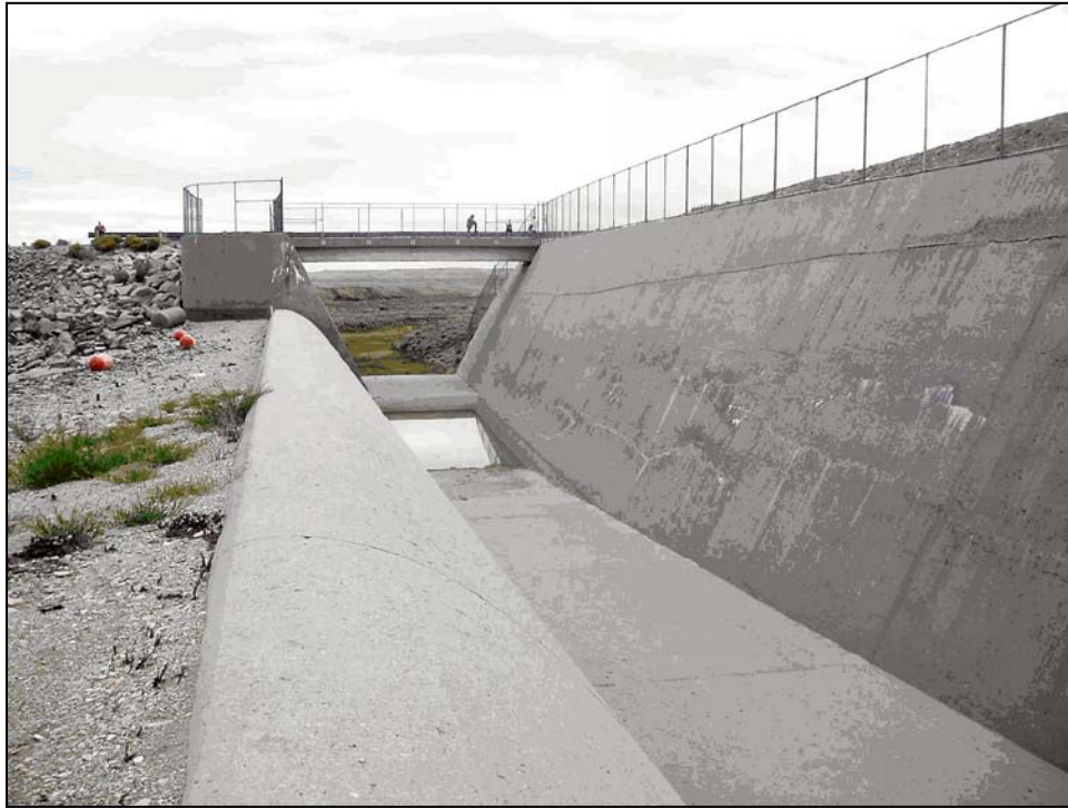
Figure 1.6.1-4. Side-channel crest (uncontrolled) spillway, Big Sandy Dam, Wyoming.
