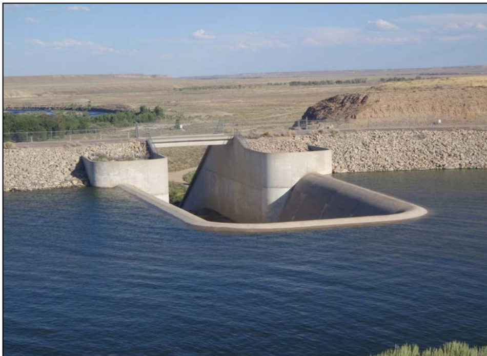
Figure 1.6.1-3. Double side-channel (bathtub) crest (uncontrolled) spillway, Fontenelle Dam, Wyoming.
