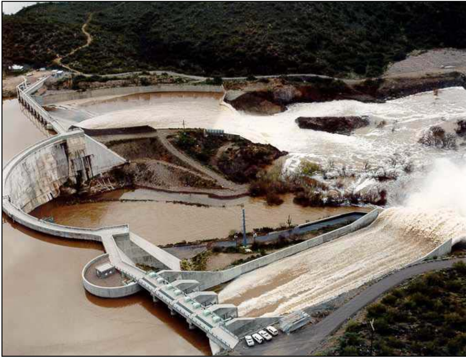
Figure 1.5.1.2-1. Example: Auxiliary spillway (gated) in foreground and service spillway (gated) in background, Stewart Mountain Dam, Arizona.
