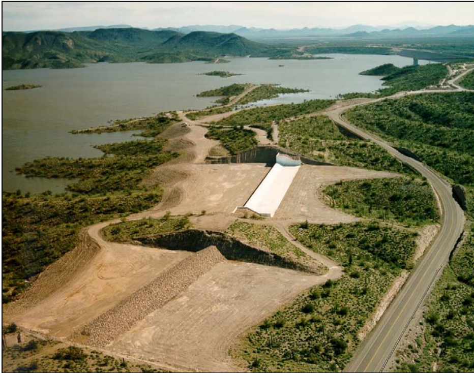
Figure 1.5.1.3-1. Example: Emergency spillway (fuseplug) in foreground and auxiliary spillway (ogee crest) in background, New Waddell Dam, Arizona.
