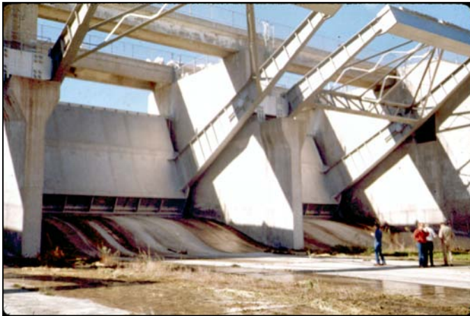
Figure 1.6.1-7. Radial gated (controlled) spillway, Bradbury Dam, California.
