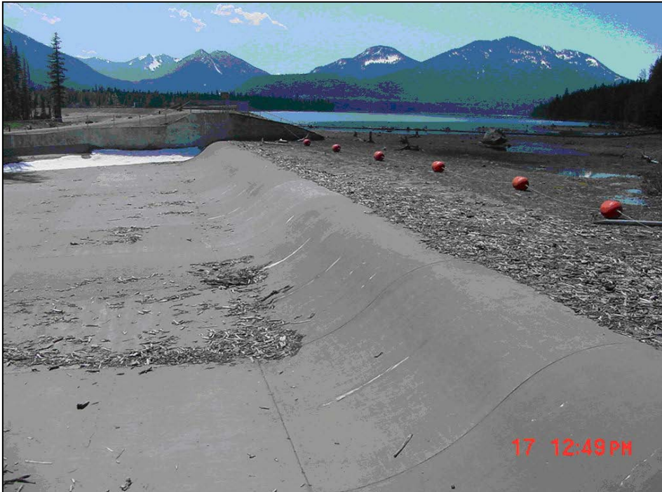
Figure 1.6.1-2. Ogee crest (uncontrolled) spillway, Bumping Lake Dam, Washington.
