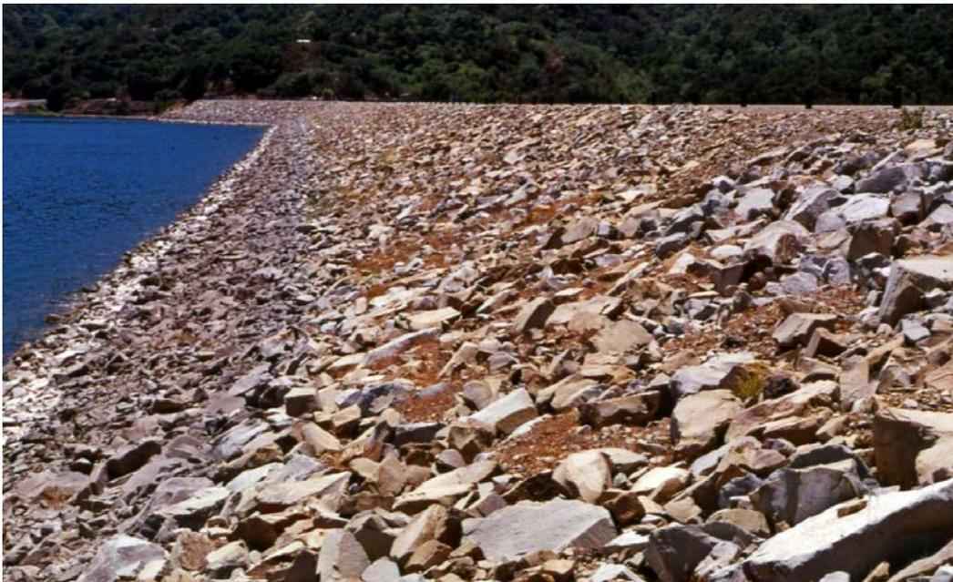
Figure 7.1.1-1. Riprap slope protection of an embankment dam.
