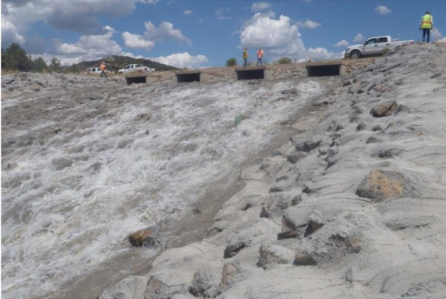
**Figure 7.5-2. Grouted riprap in drop structures downstream from Ridges Basin Dam.**
