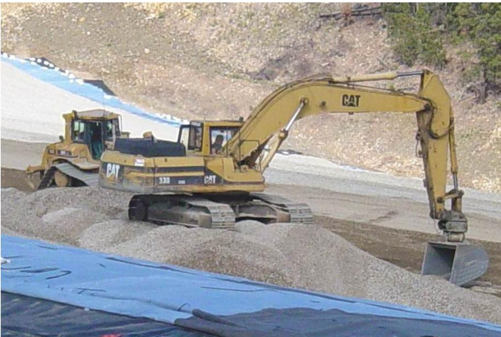
**Figure 19.6.4-2. Photograph of an excavator removing the tops of thick piles of cover material. Attempting to move such thick piles with a bulldozer is likely to damage the geotextile because of the high traction forces required to push a thick layer of material.**
