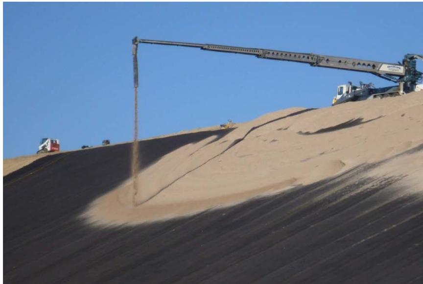
Figure RW8. Photograph showing a telescoping conveyor placing sand cover onto the geonet composite at Red Willow Dam.
