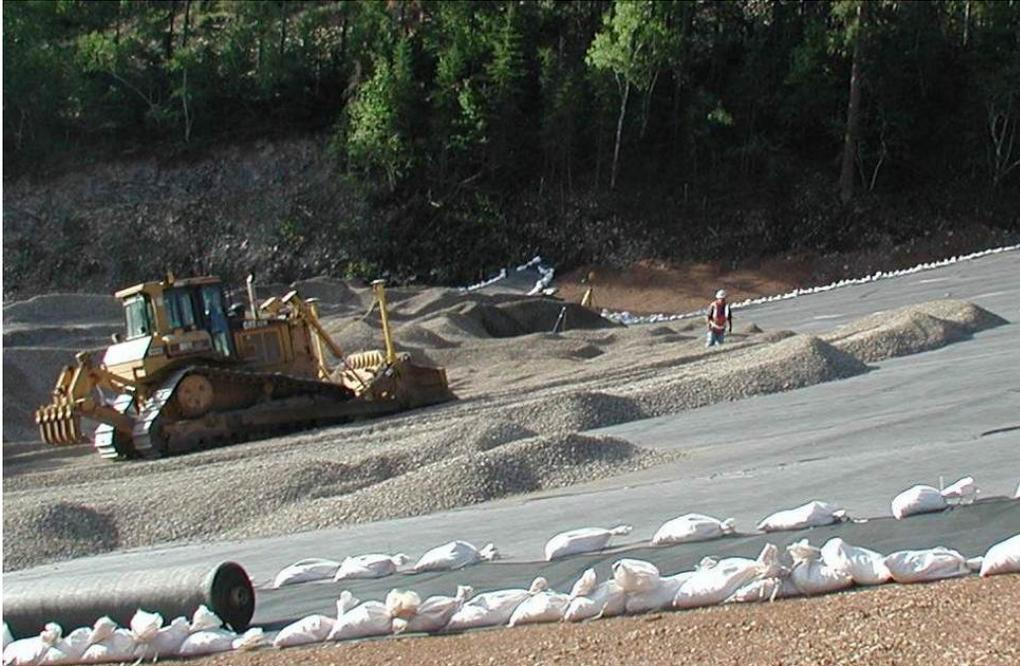
**Figure 19.6.4-3. Photograph of a low-ground-pressure bulldozer grading cover material to a uniform thickness of 1.5 feet. Note that material is pushed upslope and the presence of an inspector monitoring the work.**
