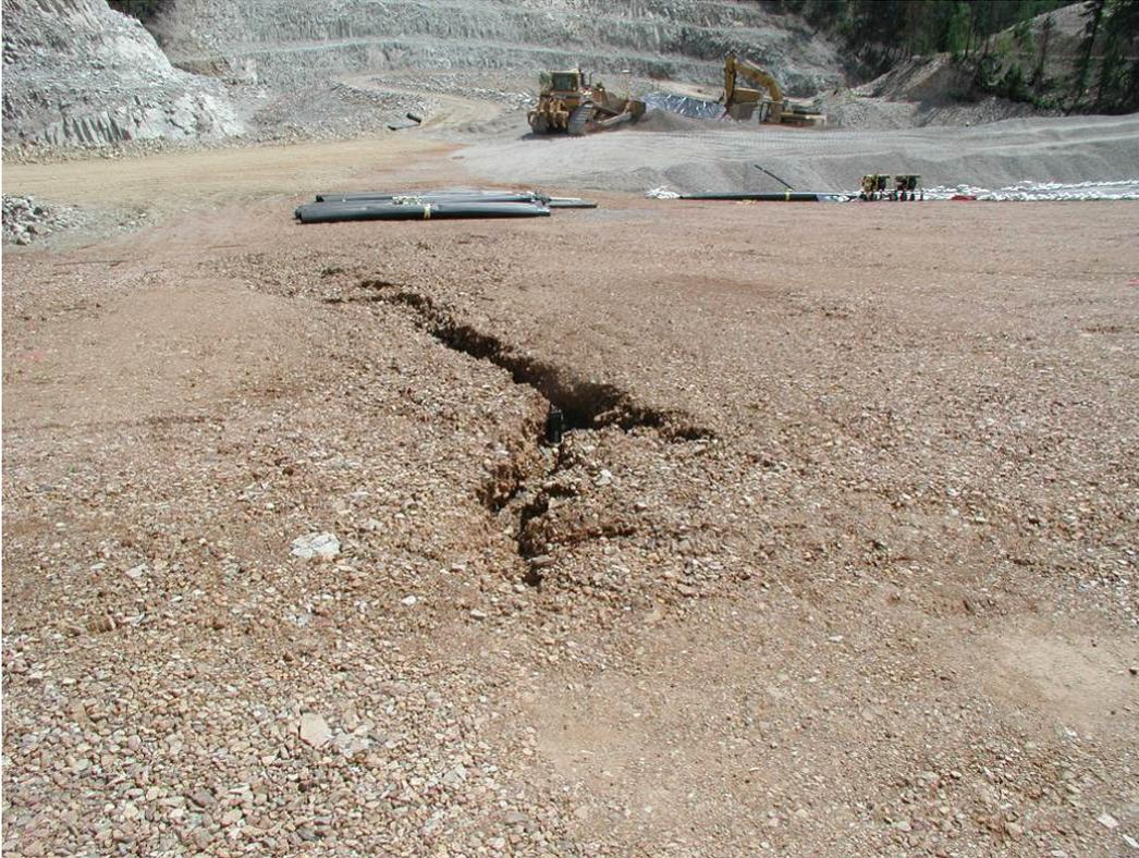
**Figure 19.6.1-2. Photograph showing a defect in a prepared subgrade surface for which the contractor wanted approval. This portion of the subgrade was rejected by the inspector and had to be filled and smoothed.**
