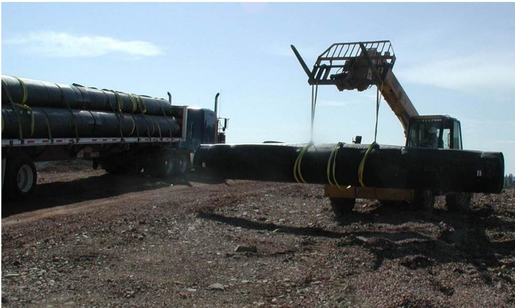
**Figure 19.5-2. Photograph showing proper offloading of geotextile product rolls. Cloth slings, rather than the forks of the lift, are used to properly unload this delivery.**
