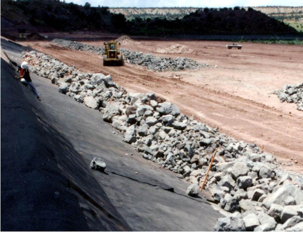
**Figure 19.6.4-5. Photograph showing riprap placement on a geotextile. The slope height that can be covered by this method is limited by the equipment reach.**
