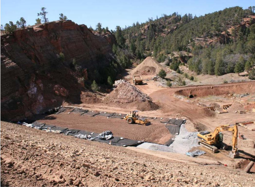
**Figure A3. Photograph showing compaction of embankment fill placed over a geotextile separation layer. View is looking down from the embankment crest.**
