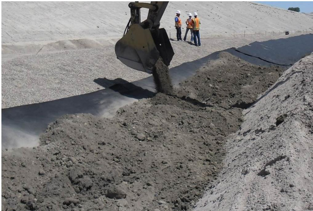
Figure RW10. Photograph showing installation of geotextile and zone 1 over the toe drain.
