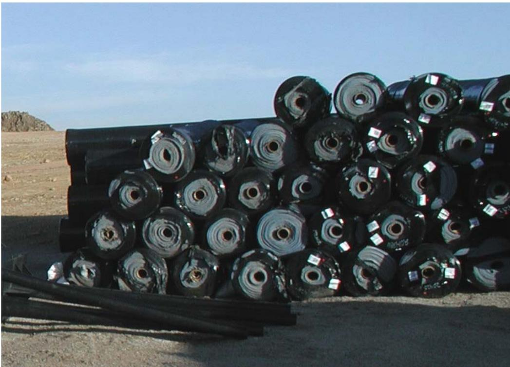
**Figure 19.5-3. Photograph of geotextile storage. A layer of fine-grained soil was placed in the storage area to avoid placing the rolls directly on the rocky soil, which is visible on the left side of the photograph. Damage to the ends of the protective wrappers is evident; the inspector required these rolls to be covered by a tarp to prevent contamination by dust and to avoid degradation from prolonged UV exposure.**
