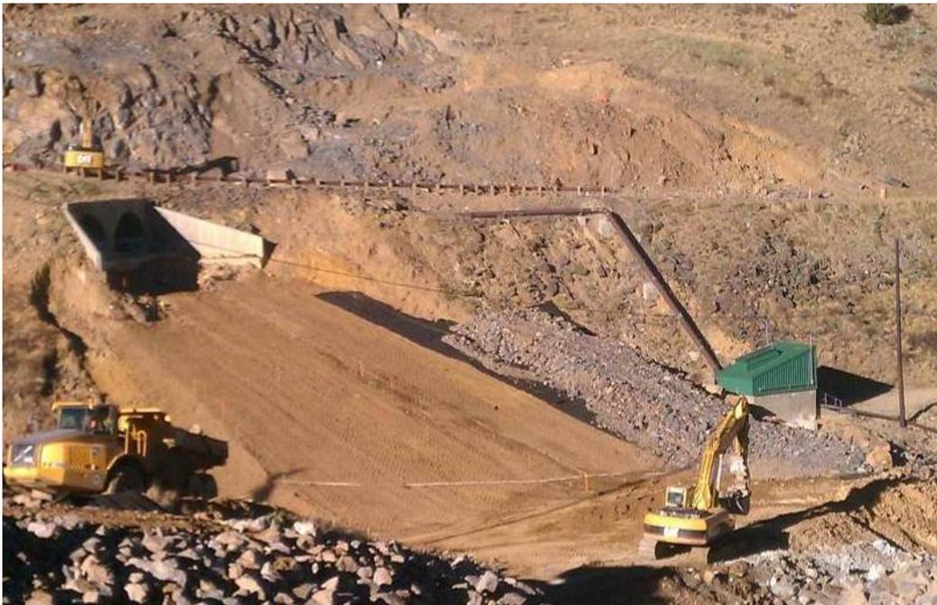
**Figure SM3. Photograph showing the flattened 3H:1V slope and initial placement of geotextile, blasted rock, geotextile, and riprap in the left channel berm on October 16, 2012.**
