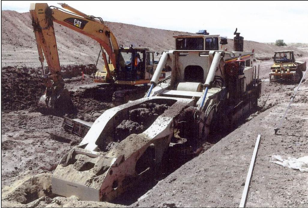
**Figure MF3. Photograph of a trenching machine excavating a trench and backfilling it with a geotextile-wrapped pipe surrounded by a sand backfill.**
