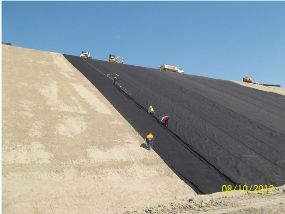
Figure RW2. Photograph showing a view of the prepared downstream surface and initial installation of geonet composite panels at Red Willow Dam.
