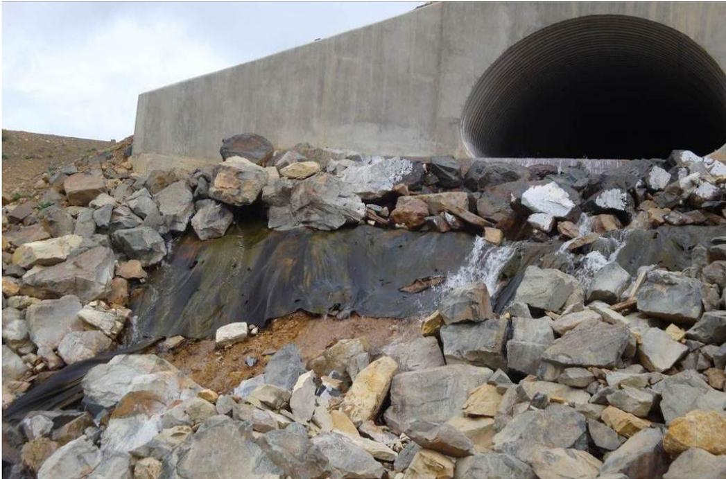
Figure SM1. Photograph showing damage to the riprap armor and underlying geotextile after a small flood event in 2010 at the Summitville Mine.
