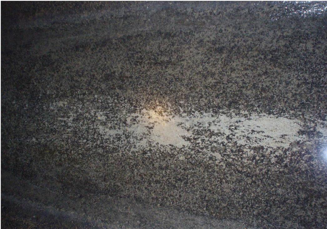
**Figure HB1.** Photograph showing sand deposits found inside the outlet works conduit.
