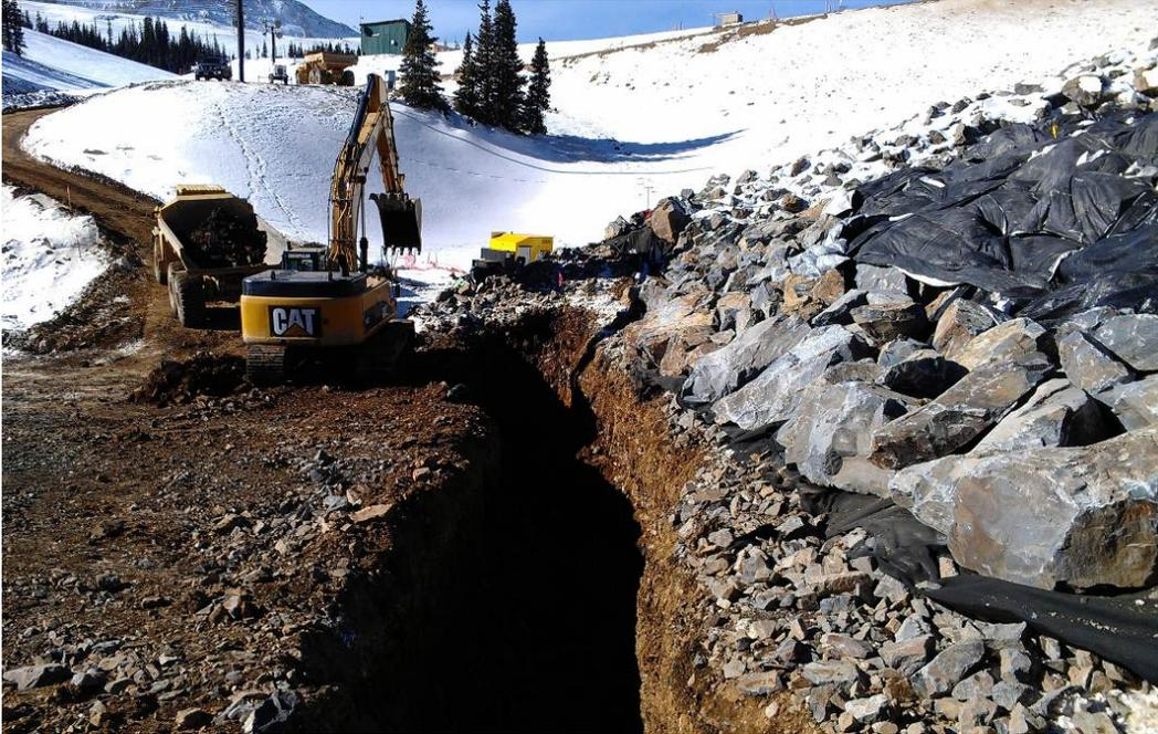
**Figure SM4.** Photograph showing excavation of the lower cutoff trench at the toe of the grouted riprap slope. The blasted rock underdrain is visible underneath the geotextile fabric in the lower right portion of the photograph.
