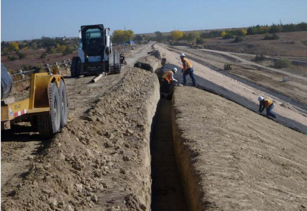
**Figure 19.6.2-2. Photograph of an anchor trench at a dam for a geonet composite.**
