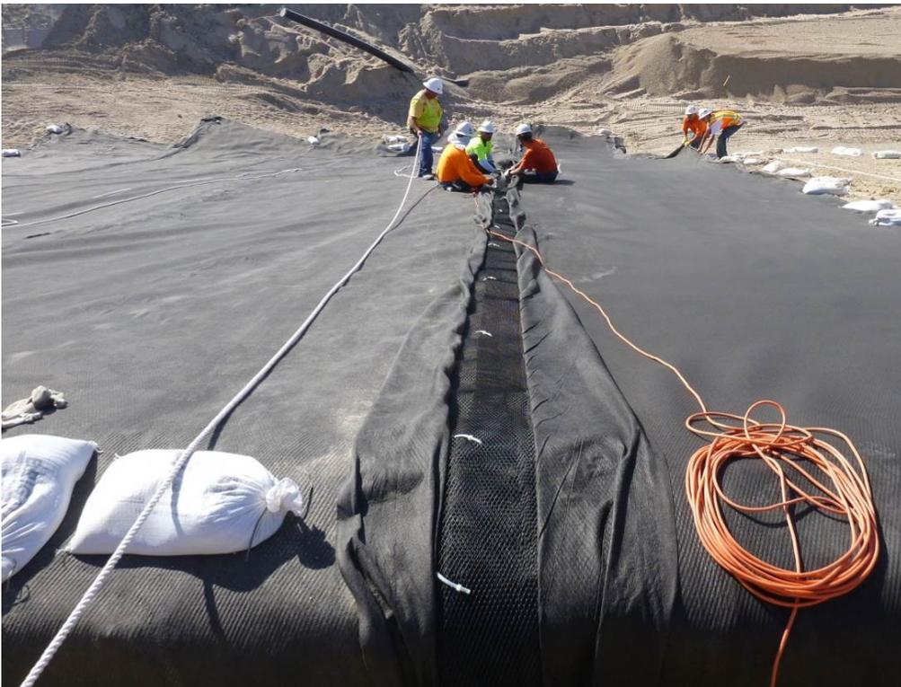
Figure RW5. Photograph showing the use of nylon ties to join the geonet layer of the composite.
