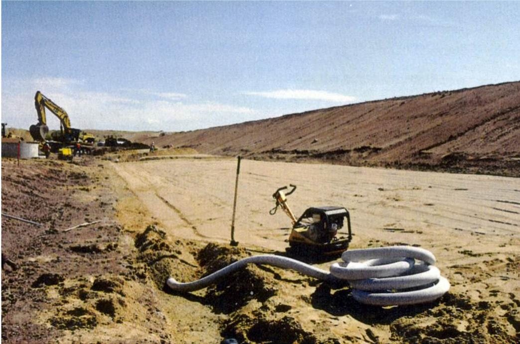
**Figure MF5.** Photograph of a geotextile-wrapped pipe emerging from a completed segment of the Many Farms Dam toe drain trench.
