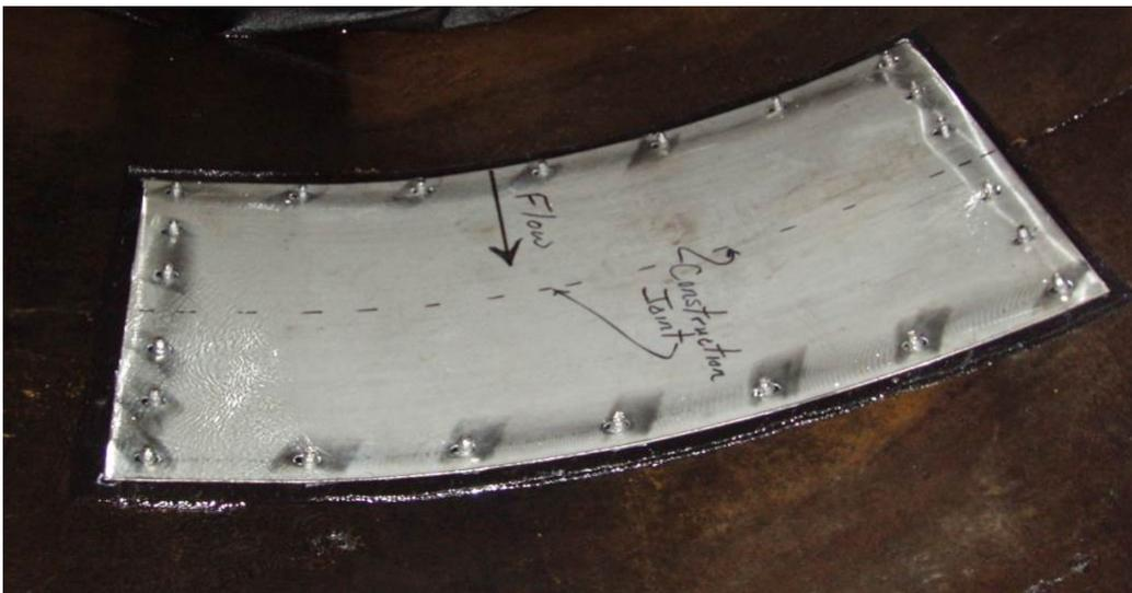
Figure HB5. Photograph showing the nuts have been tightened down to complete the installation of the cover plate and underlying geotextile filter.
