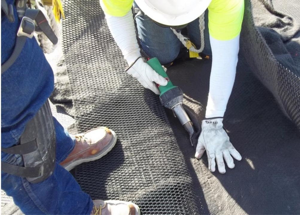
Figure RW4. Photograph showing a closeup view of the heat bonding of a seam in the lower 16 oz/yd<sup>2</sup> geotextile in the geonet composite.
