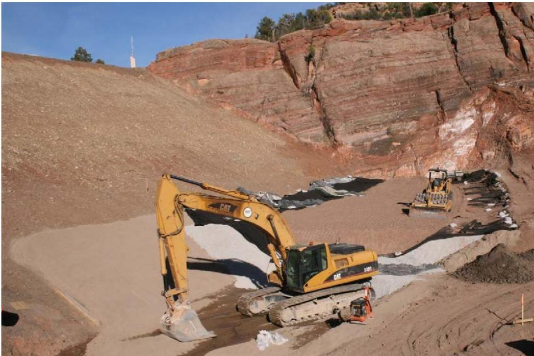
**Figure A2. Photograph showing placement of sand filter (underneath excavator and partially up embankment slope), gravel drain (light-colored material), geotextile (black-colored material), and new embankment fill.**
