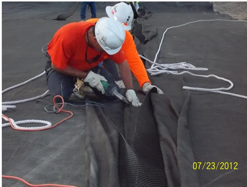
Figure RW3. Photograph showing heat bonding a seam in the lower 16 oz/yd<sup>2</sup> geotextile in the geonet composite.
