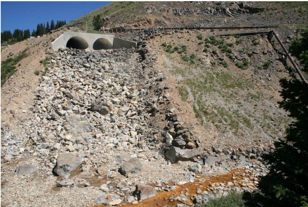
Figure SM2. Photograph showing an overview of the "Run-down" as it appeared in the summer of 2012 after some repair and addition of riprap. This is the 2H:1V channel that Reclamation was asked to evaluate.
