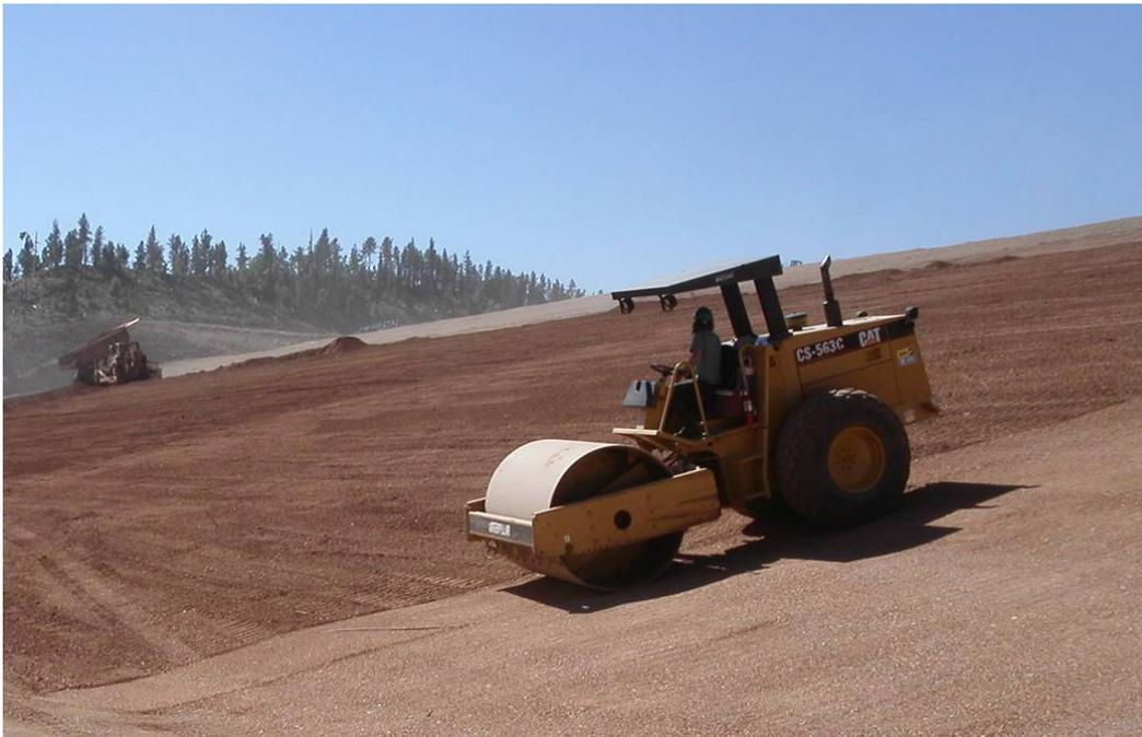
**Figure 19.6.1-1. Photograph showing compaction equipment preparing a suitably smooth and firm subgrade surface for geotextile placement.**
