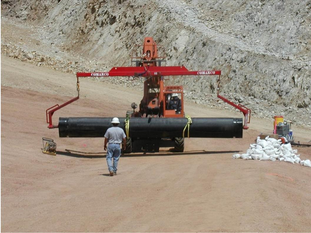
**Figure 19.6.2-1. Photograph showing how a geosynthetic roll is moved with a pipe, spreader bar, and a spotter. The spotter (person walking in front of the equipment) is needed to ensure that the geosynthetic product does not strike any other objects that could damage the material.**
