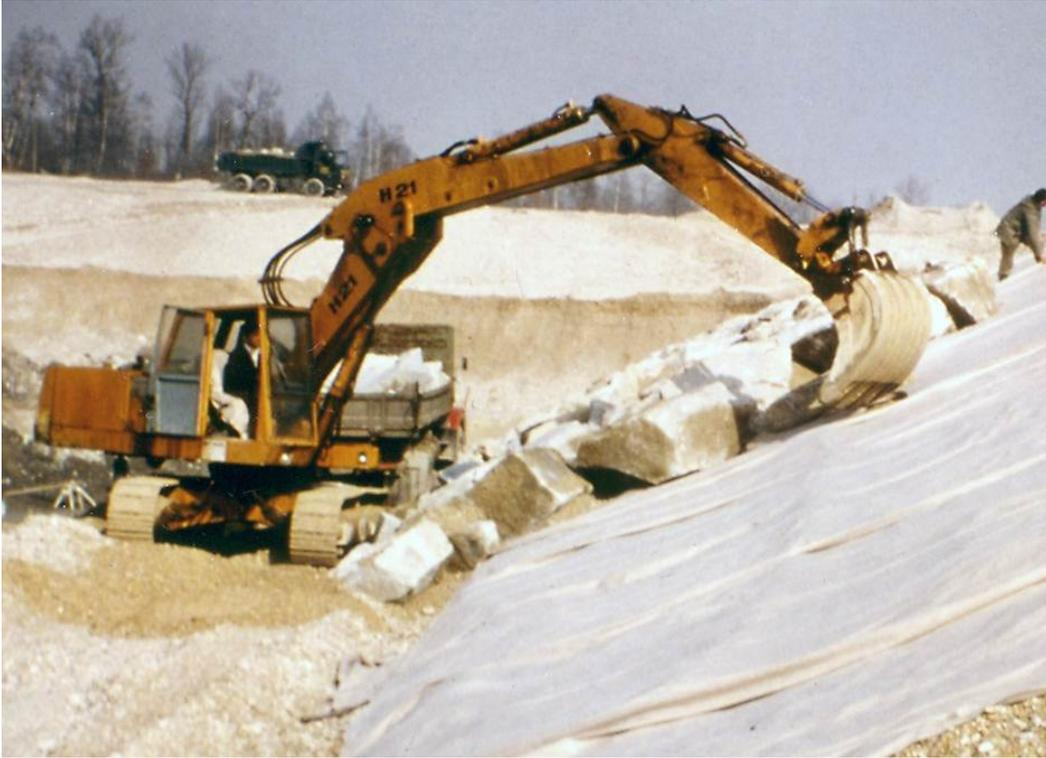
Figure 19.6.4-6. Photograph showing placement of large riprap as slope protection. Note that a layer of bedding soil has been placed as a cushion under each piece of riprap prior to gently placing the large rock into position.
