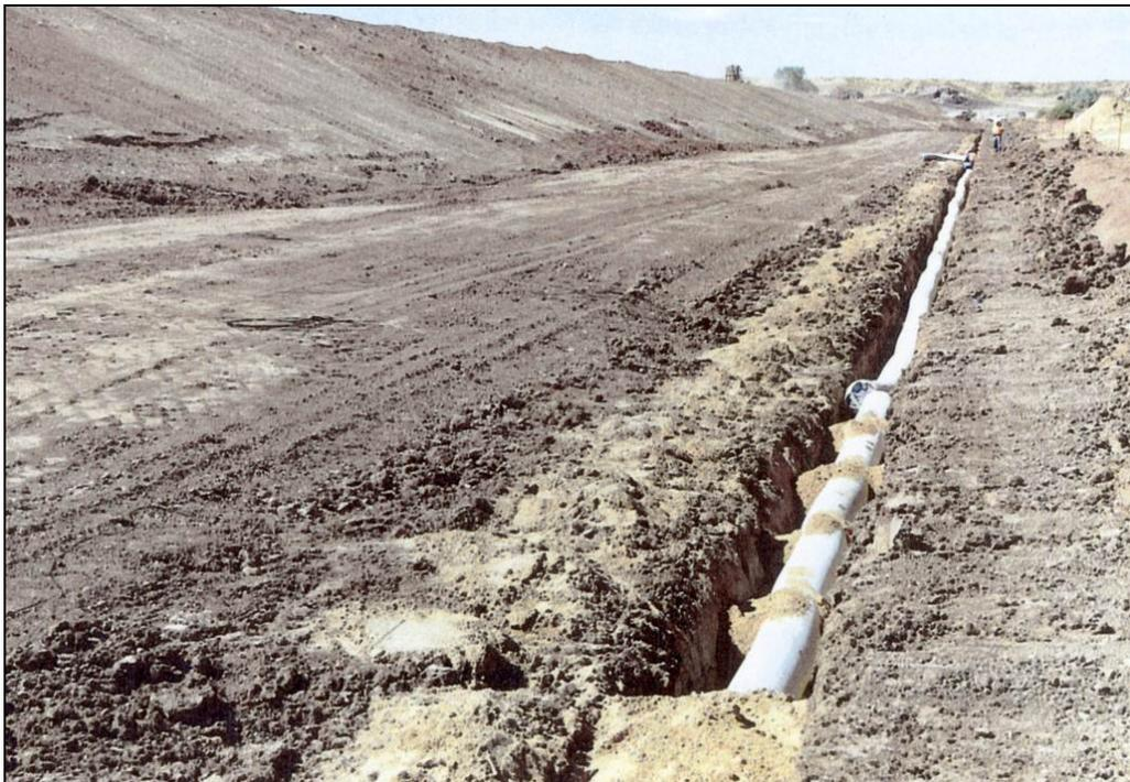
**Figure MF4. Photograph of the toe drain trench showing geotextile-wrapped pipe without sand backfill. The trenching machine was so efficient that sand deliveries to the site could not keep up with pipe installation rates.**
