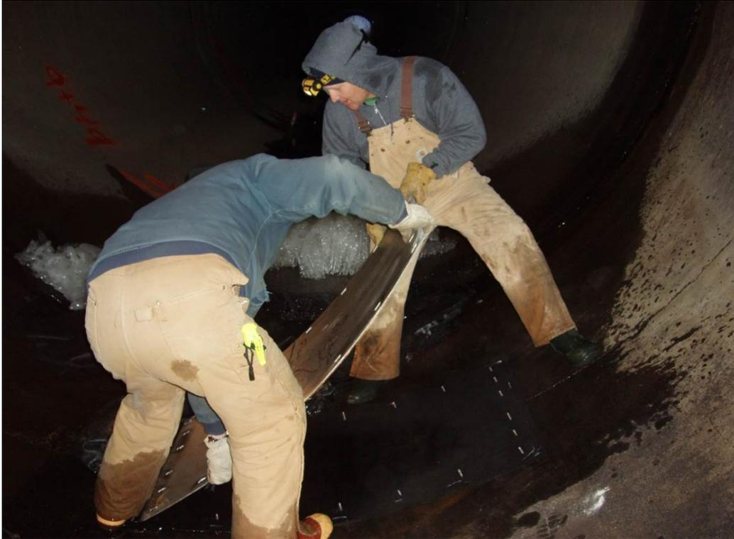
Figure HB4. Photograph showing workers lowering the cover plate into place.
