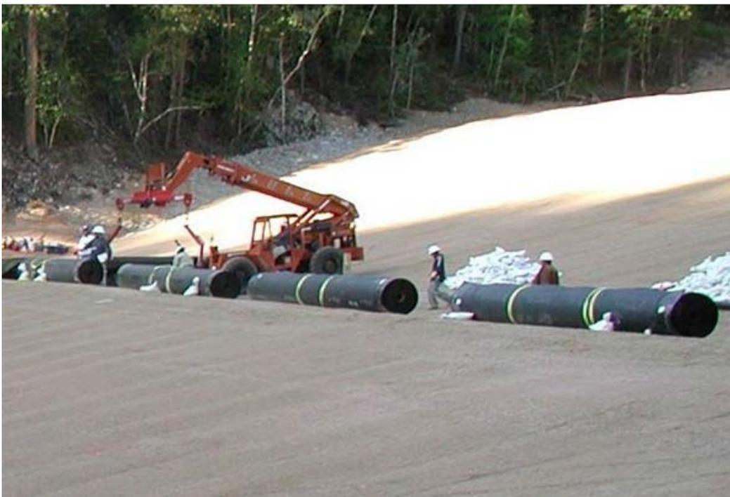
**Figure 19.6.2-3. Photograph showing a bench used to divide a long slope and provide an intermediate anchor location. Note the presence of proper equipment, sufficient labor, and adequate supplies.**
