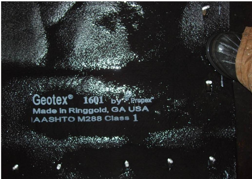
Figure HB3. Photograph showing two layers of geotextile having been placed over the conduit joint and anchor bolts.
