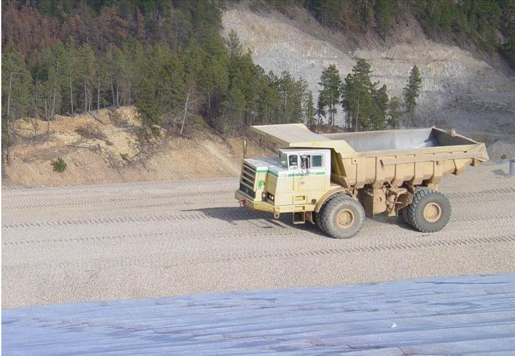
**Figure 19.6.4-1. Photograph showing a haul road where the cover layer thickness has been temporarily increased to 5 feet to protect the geotextile from heavy equipment loading.**
