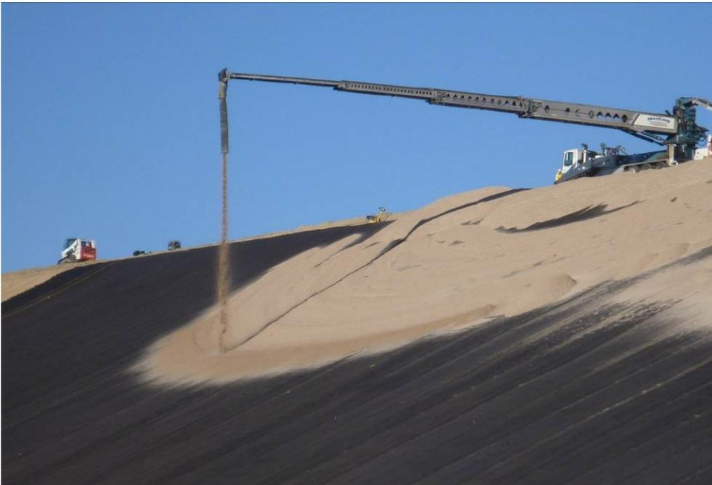
**Figure 19.6.4-4. Photograph showing initial placement of sand cover onto a geonet composite using a telescoping conveyor at Red Willow Dam in 2012. Note that placing cover from upslope to downslope is usually not allowed; use of other types of equipment in a downslope manner would damage the geotextile.**
