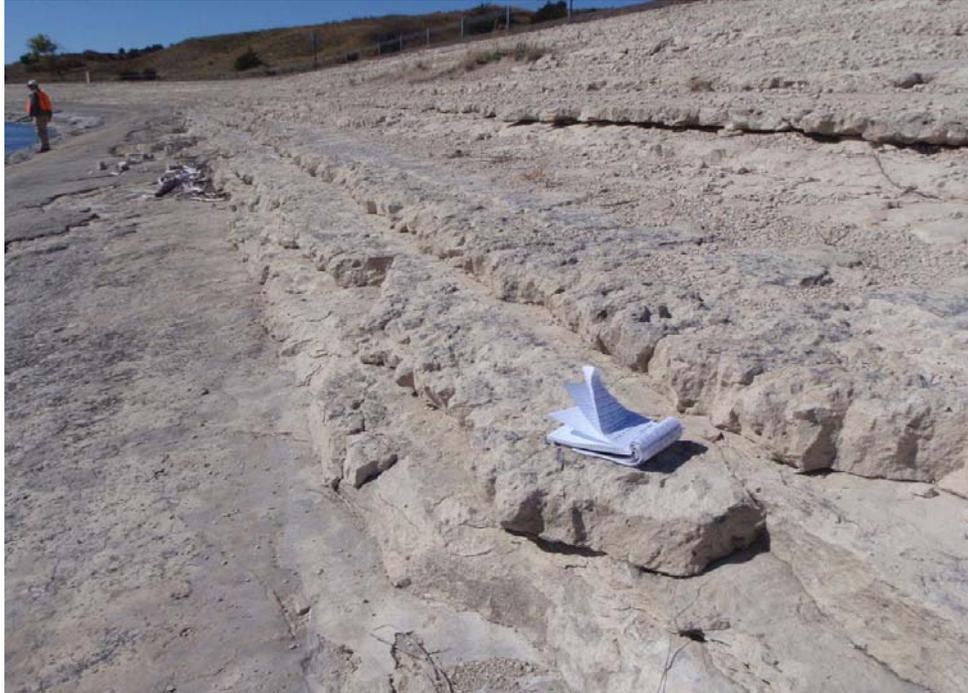
**Figure 17.2.2-5. Typical condition of upstream slope protection at Merritt Dam, Nebraska.**
