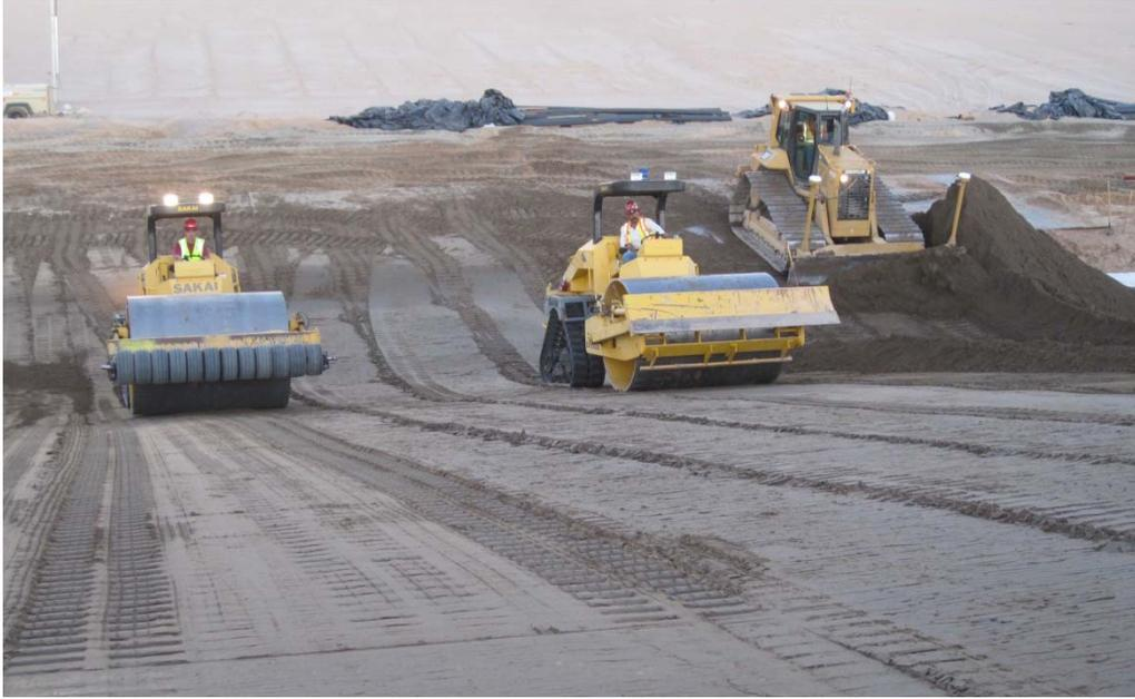
**Figure 17.6.3-1. Plating soil-cement placement at Warren H. Brock Reservoir, California.**
