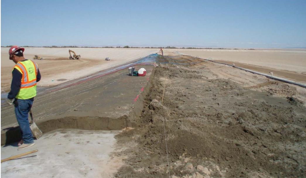
**Figure 17.5.5-2. Plating soil-cement placement at Warren H. Brock Reservoir, California. (Note the vertical construction joint.)**
