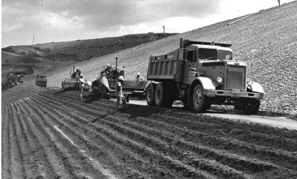
Figure 17.6.3-2. Placement of soil-cement slope protection, Starvation Dam, Utah.
