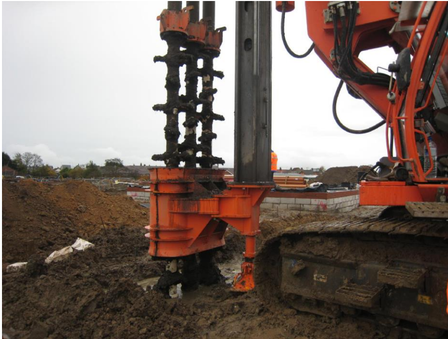
Figure 16.11.1-2. Deep soil mixing (multiple augers).
