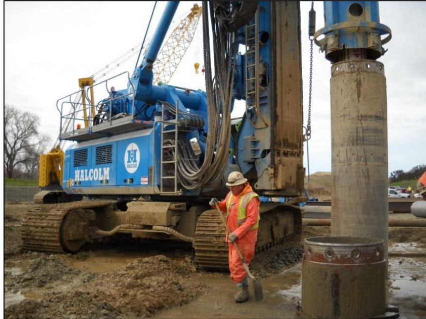
Figure 16.10.1-2. Drill bit used for installation of secant pile cutoff wall (Mormon Island Auxiliary Dam, California).
