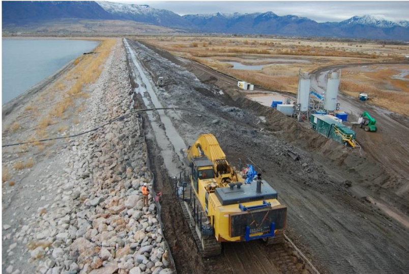
Figure 16.5.5-1. Continuous excavation of CB cutoff wall (A.V. Watkins Dam, Utah).
