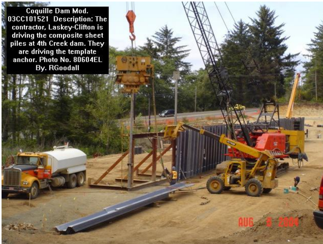
Figure 16.9-1. Installation of sheet pile cutoff wall (Coquille Dam, Oregon).
