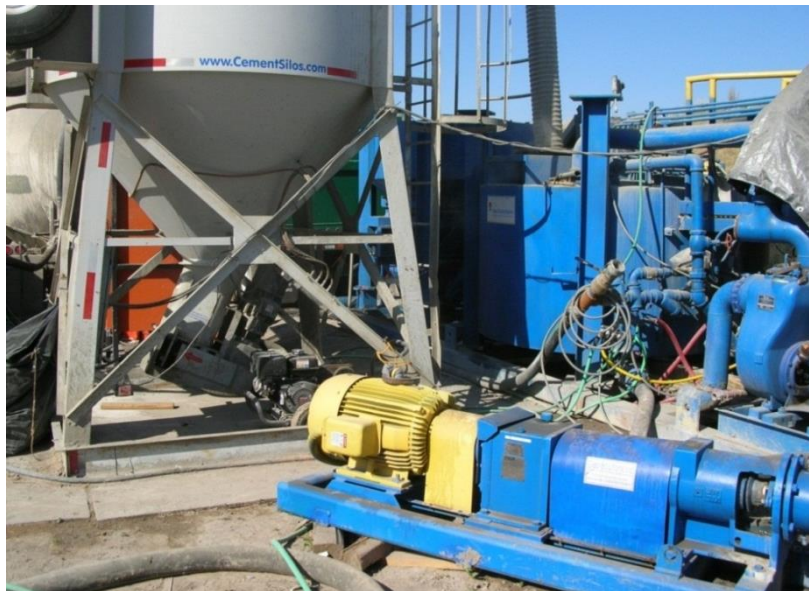
Figure 16.5.5-2. CB mixing plant (A.V. Watkins Dam, Utah).
