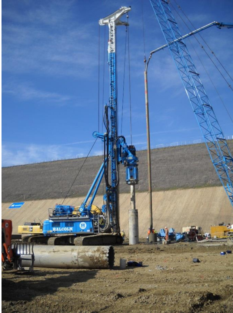
Figure 16.10.2-1. Tremie backfilling of secant piles (Mormon Island Auxiliary Dam, California).
