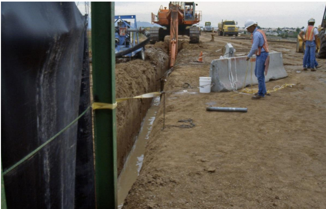
Figure 16.8.2-1. Biopolymer slurry trench (Reach 11 Dikes, Arizona).
