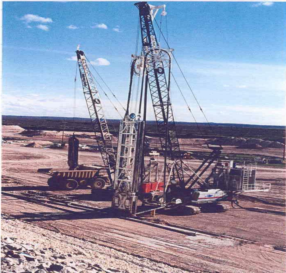
Figure 16.6-2. Rockmill, clamshell, excavating the SCB cutoff wall (Twin Buttes Dam, Texas).
