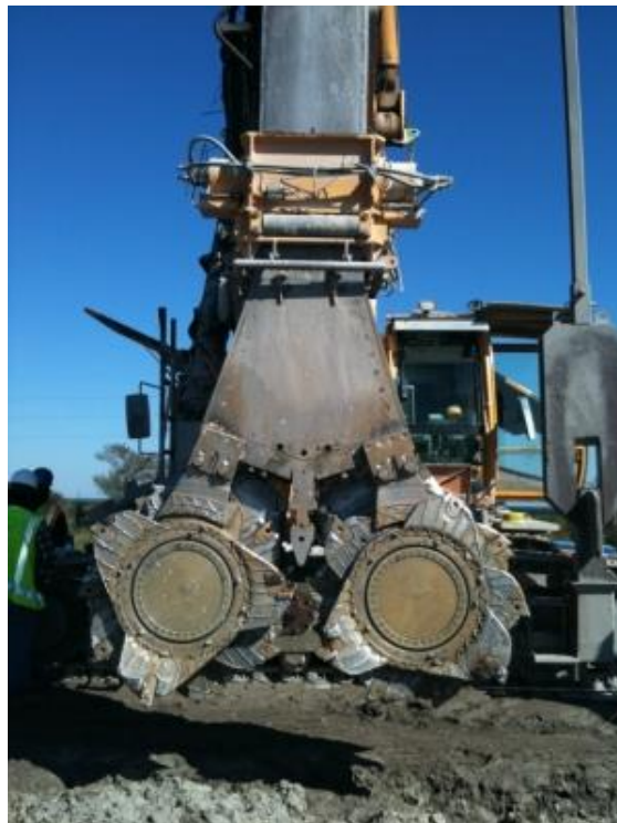
Figure 16.11.1-3. Deep soil mixing.
