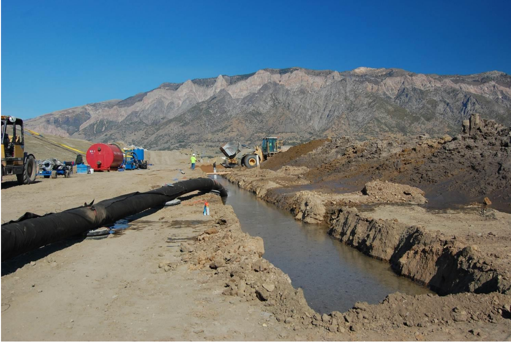
Figure 16.8.2-2. Biopolymer slurry trench (A.V. Watkins Dam, Utah).
