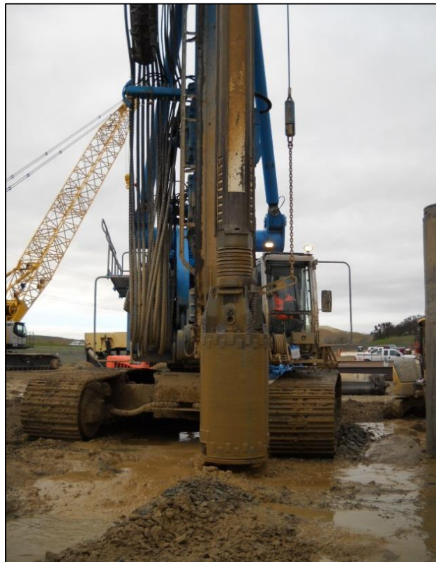
Figure 16.10.1-3. Installation of secant pile cutoff wall (Mormon Island Auxiliary Dam, California).
