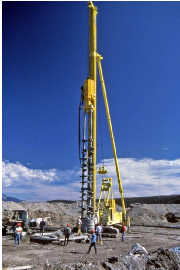
Figure 16.11.1-1. Deep soil mixing auger system (Jackson Lake Dam, Wyoming).
