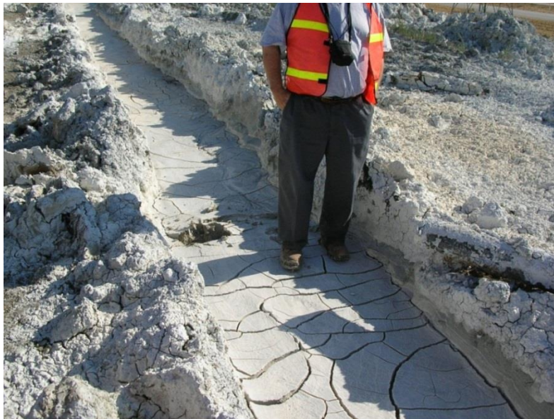
Figure 16.5.5-4. CB cutoff wall after initial set (A.V. Watkins Dam, Utah).
