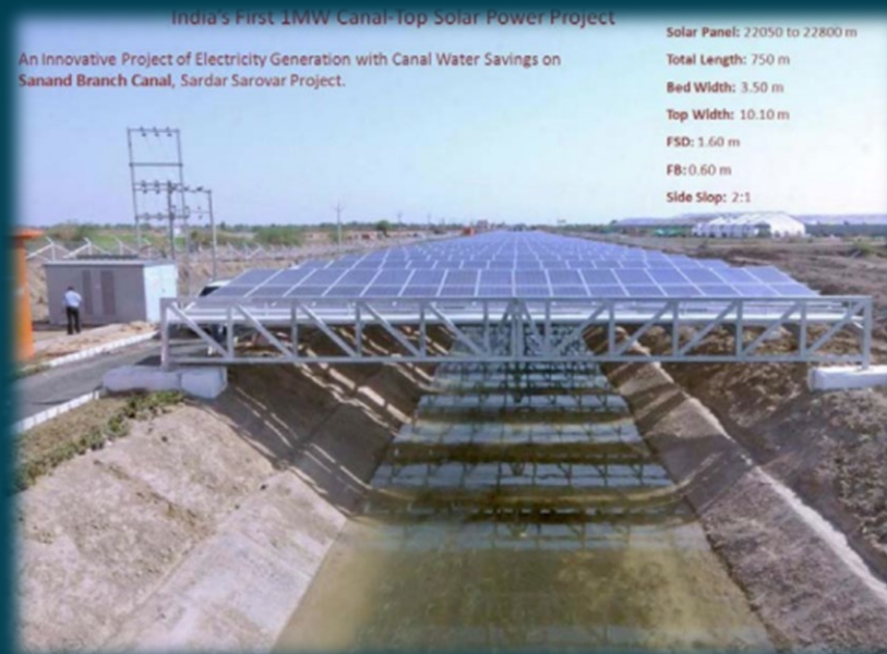
One of the early solar panel projects in Gujarat, India.
