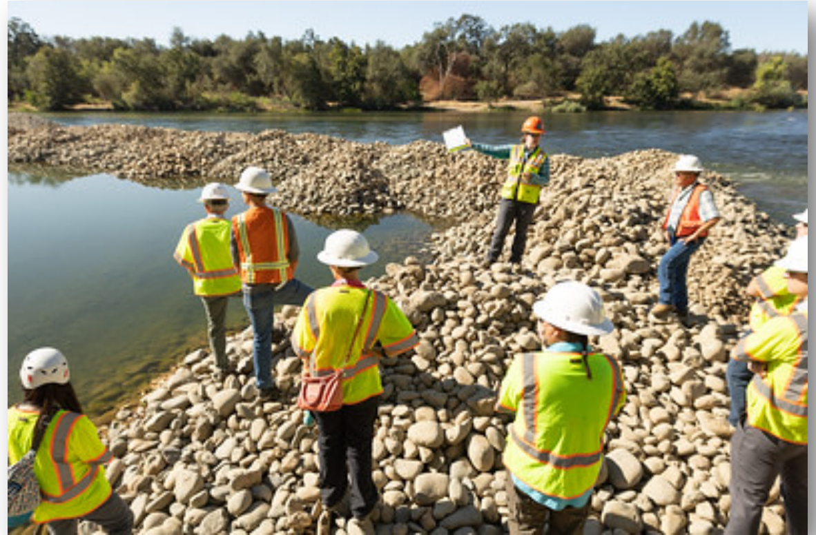
Photo: Installation of the Sailor Bar Project, an instream gravel bar complex to create habitat for native Chinook Salmon in the Lower American River in Sacramento, California.
