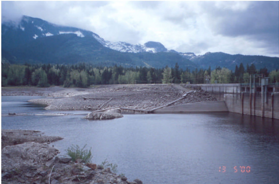
Cheakamus Dam (British Columbia Hydro and Power Authority)
