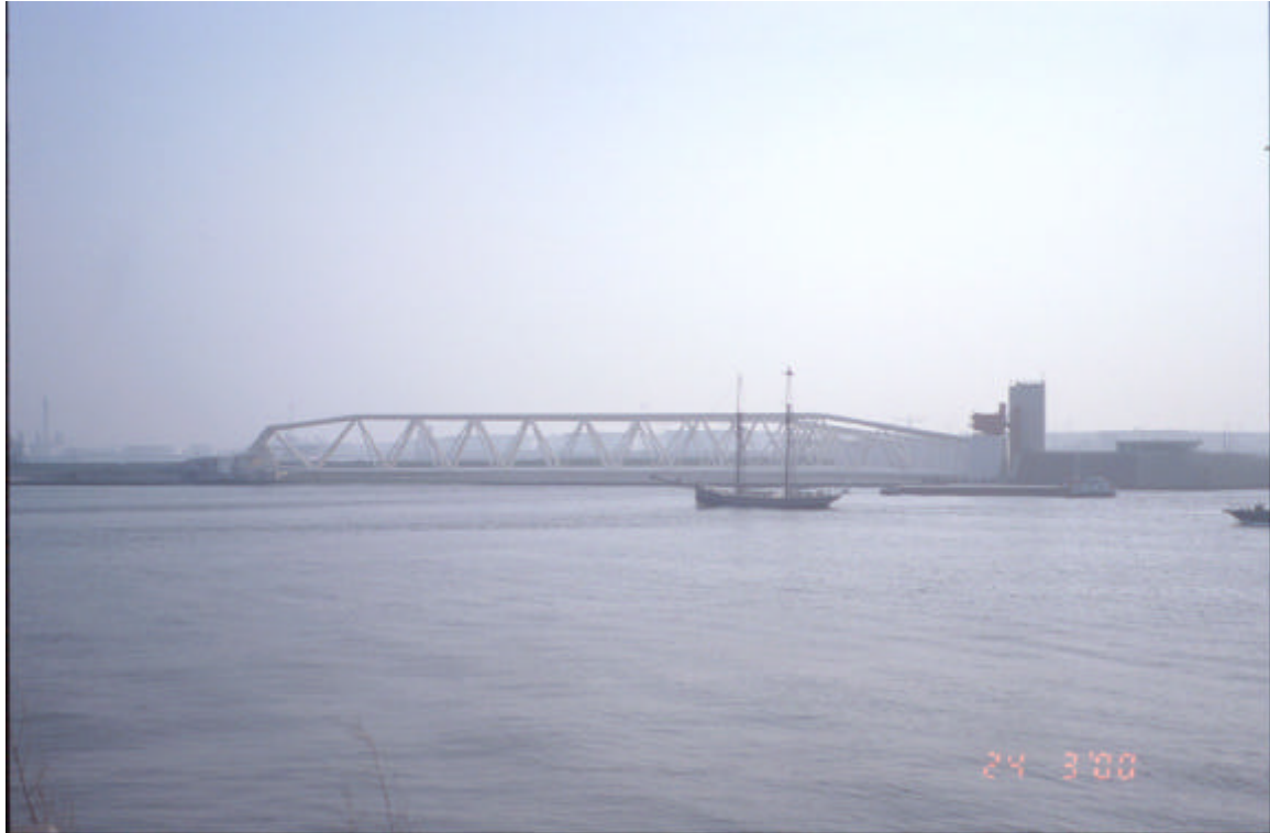
New Waterway Storm Surge Barrier Rotterdam (Ministry of Transport, Public Works and Water Management)
