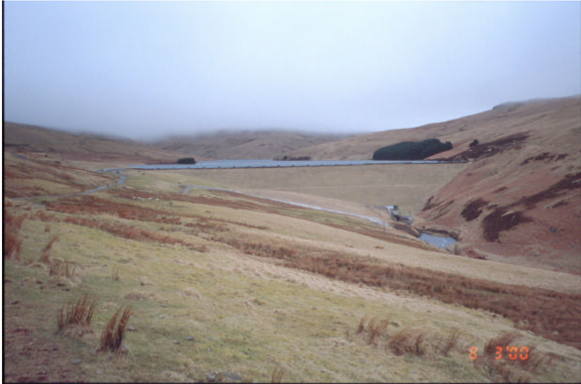
Upper Glendevon Dam Scotland (Scottish and Southern Energy)
