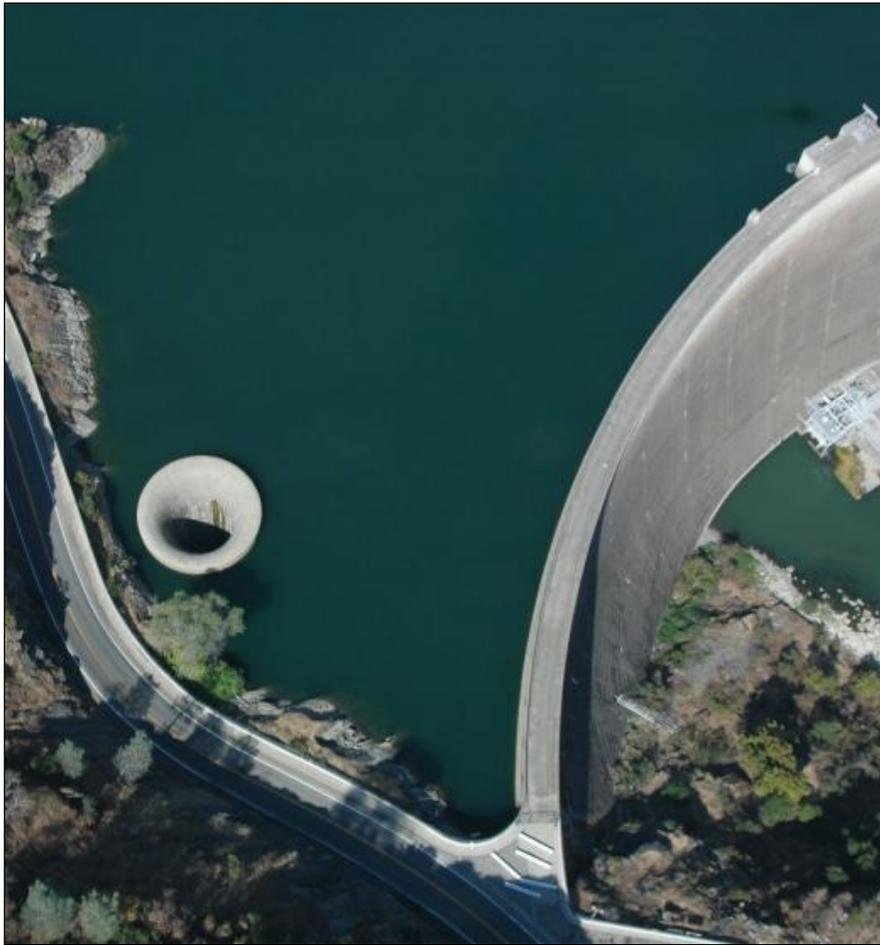
Figure G-2-2.—Morning Glory Spillway, Monticello Dam (California, Reclamation).
