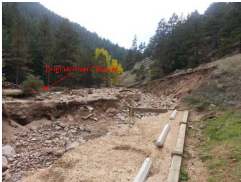
FIGURE 4.5: FOURMILE CANYON CREEK NEAR THE ENTRANCE TO THE ANNE U. WHITE TRAILHEAD NEAR BOULDER, CO. THE RED ARROW INDICATES THE PRE-FLOOD LOCATION OF THE RIVER CHANNEL.
