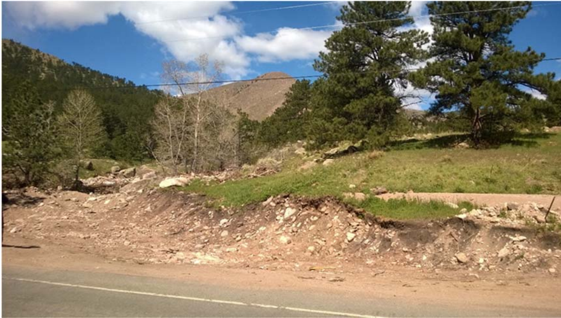
FIGURE 4.4: LEFT HAND CREEK, APPROXIMATELY 1.5 MILES UPSTREAM OF HWY 7. A DEBRIS FLOW GENERATED ON THE LEFT HILLSLOPE CROSSED THE ROAD ENTERING THE RIVER CHANNEL LOCATED ON THE OPPOSITE SIDE OF THE VALLEY.
