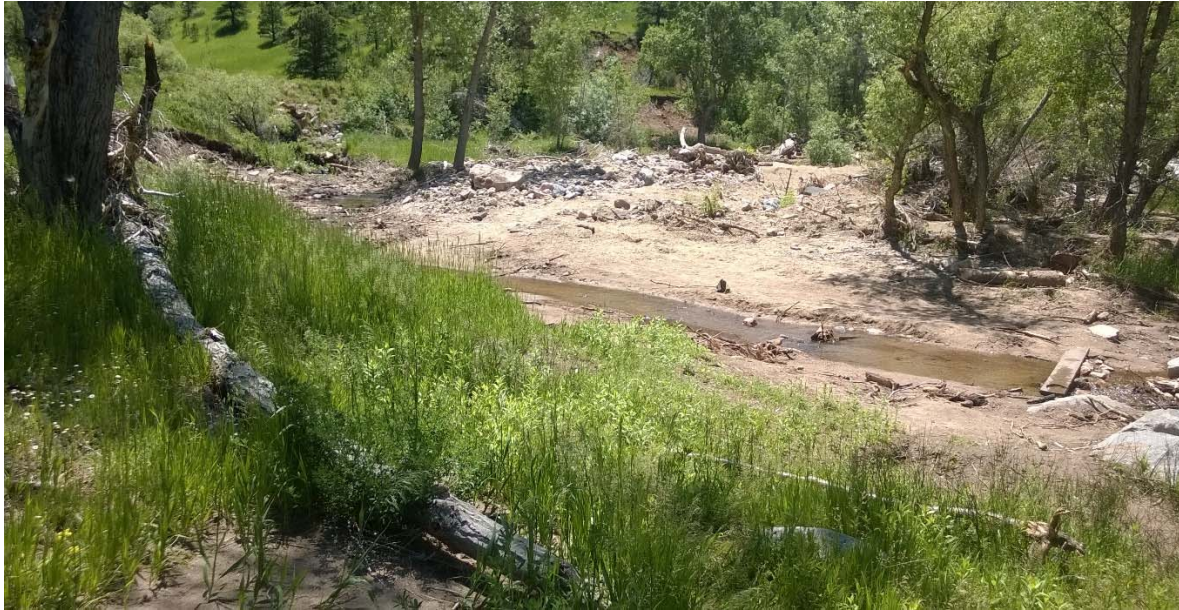
FIGURE 3.19: T1 SURFACE NEAR THE CONFLUENCE WITH SIX MILE CREEK. FLOTSAMS AND LARGE WOODEN DEBRIS FROM THE 2013 FLOOD EVENT ARE DEPOSITED ON THE WIDEN AND ERODED RIVER CHANNEL.
