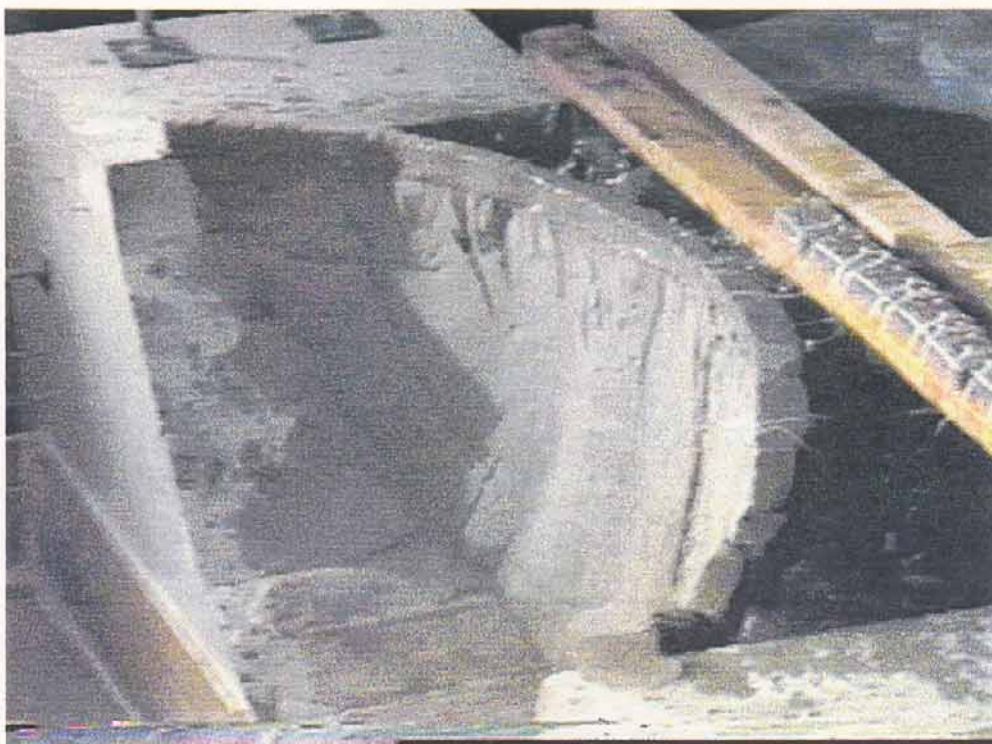
Model M11 -- 8/22/00 North view, initial cracking
