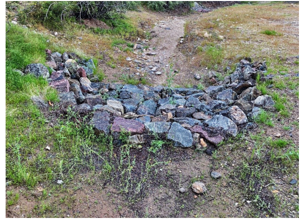
Grade control structure installed at BSA HSP site.
