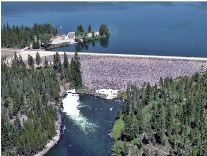
Island Park Dam, Idaho.
