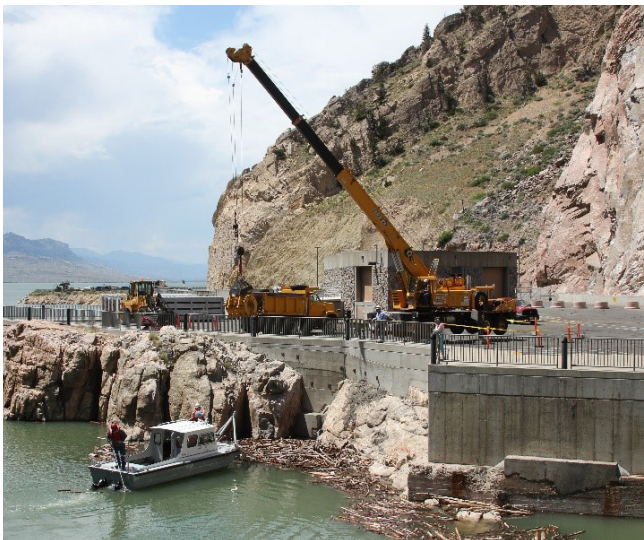
Debris removal at Buffalo Bill Dam, WY.
