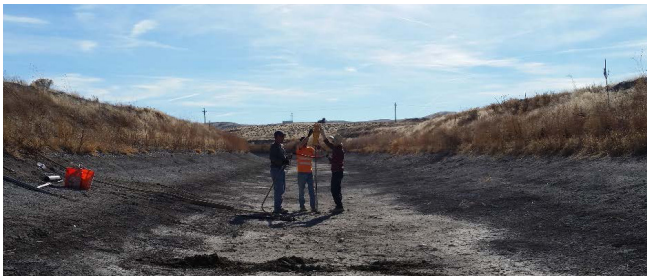
Installing field equipment in the Truckee Canal outside of Reno, Nevada.
