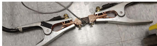
500 A to 50 mV shunt in primary circuit, part of the optical current transformer test set up.
