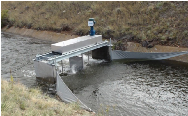
Hydrokinetic unit in operation with temporary upstream transitions made of tarps.
