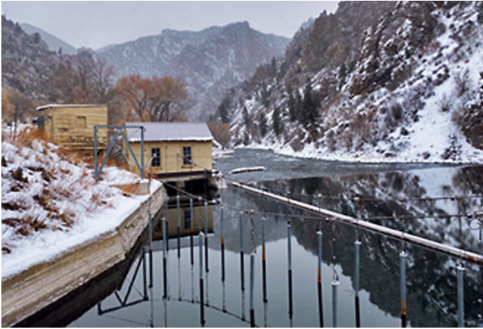
Photos of the electric fish barrier installed at the East Portal of Gunnison Tunnel in Colorado. Both photos are taken from the location of the slide gate at the inlet of the tunnel.
