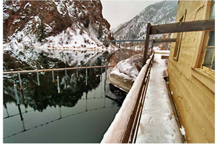
Photos of the electric fish barrier installed at the East Portal of Gunnison Tunnel in Colorado. Both photos are taken from the location of the slide gate at the inlet of the tunnel.
