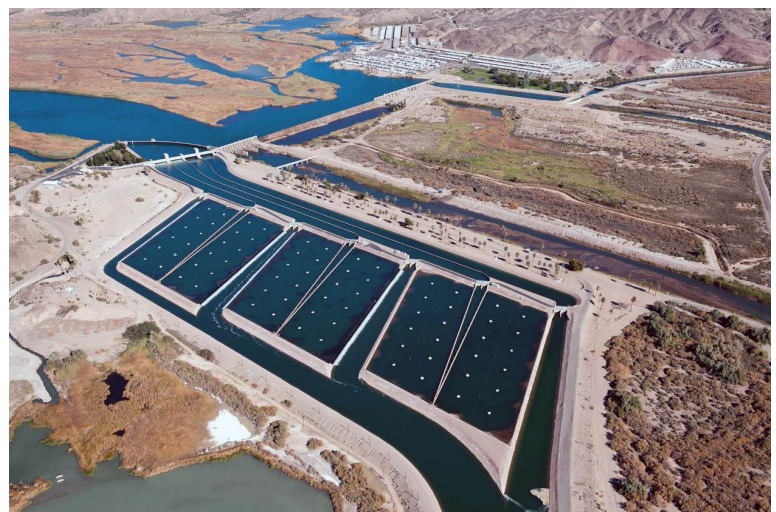
Imperial Dam and the All-American Canal System near Yuma, Arizona.
