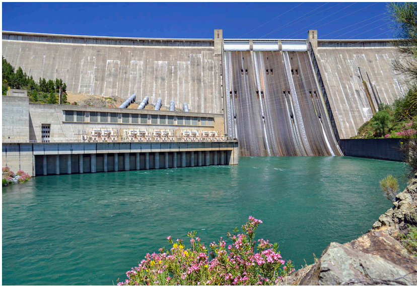
Shasta Dam and Powerplant, California.
