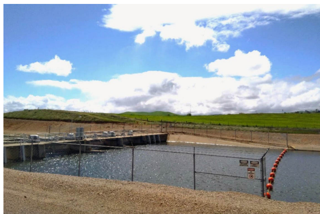
Delta Mendota Canal at milepost 64 near Santa Nella, California. (photo credit Laurel Dodgen)
