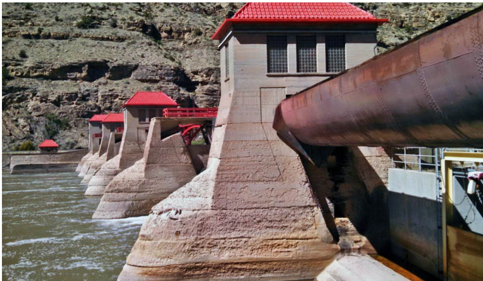
Grand Valley Diversion Dam, Colorado River, Colorado.
