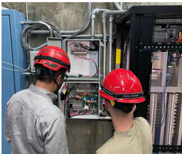
Engineers inspect instrumentation.
