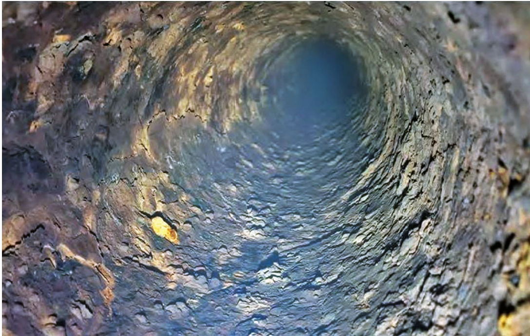
Small diameter pipe interior showing the entire surface corroded with large rust nodules.
