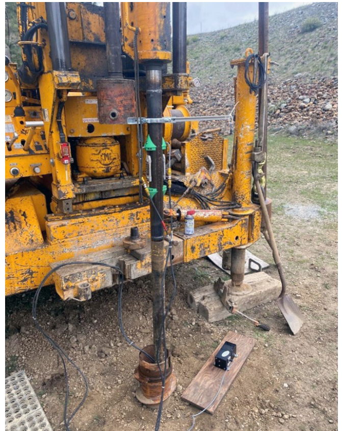
Reclamation instrumented drill rig, a CME 850, at Conconully Dam, Washington.
