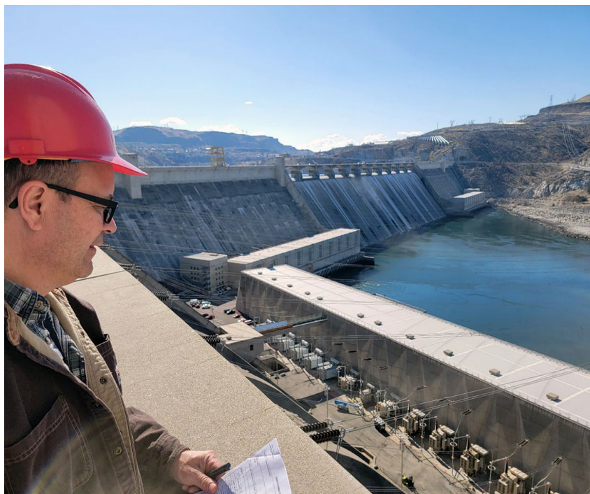
Researcher at Grand Coulee Dam.
