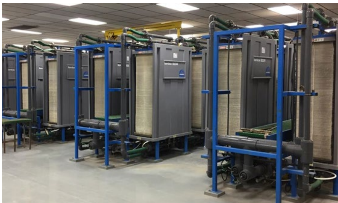
Membrane and spacer stacks for electrodialysis.
