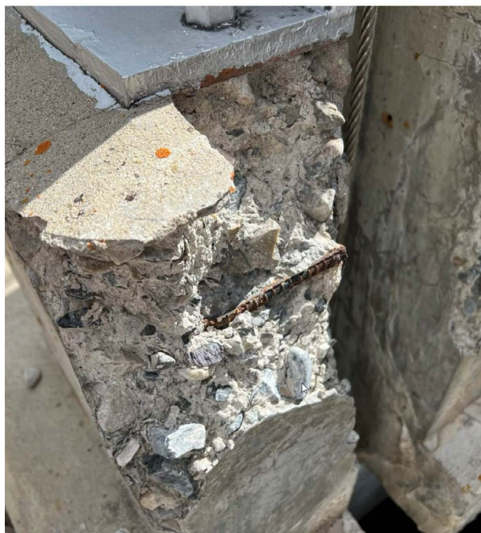
Spalling pedestal with exposed reinforcing steel.
