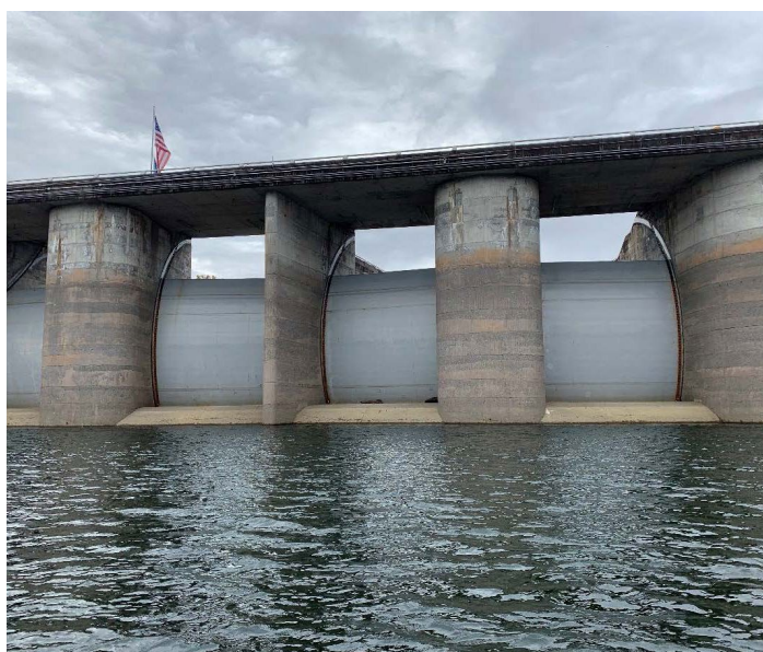
Radial gates coated with polysiloxane at Fontana Dam, North Carolina.
