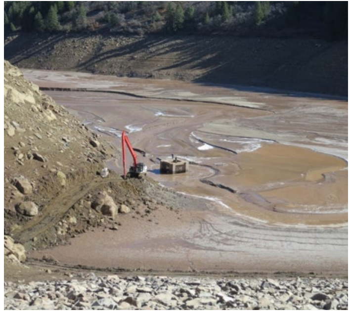
Paonia Reservoir outlet works intake structure during emergency actions to maintain diversion.
