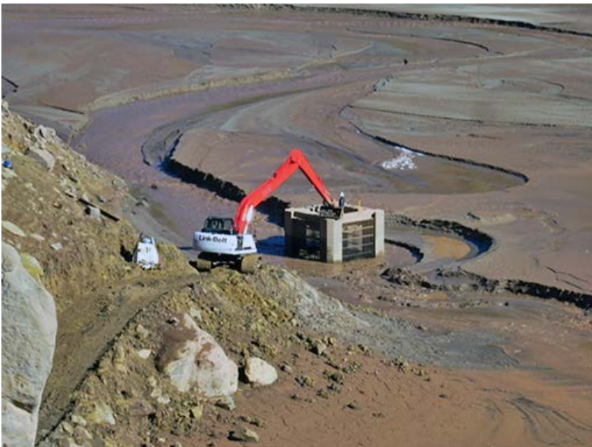
Figure 14. Looking at sedimentation at Paonia Reservoir that affects intake operations and storage capacity. Reservoir sediment management research could help develop solutions.
