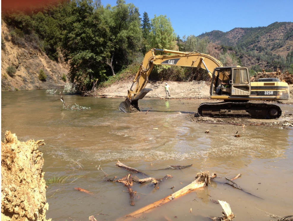
Figure 18. Research is needed to improve capability to predict river response from constructed habitat features such as this example of a log jam being constructed on the Trinity River. Photograph courtesy of Nate Bradley, Reclamation.
