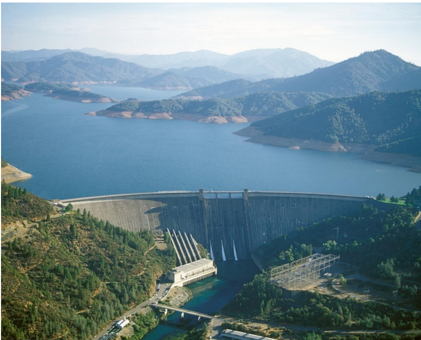
Figure 17. Shasta Dam on the Sacramento River (CA) where high-head fish passage research could help provide future fish passage options.
