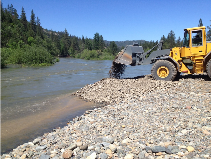
Figure 13. Research is needed to understand timing and ecological benefits of gravel augmentation downstream of Reclamation facilities that have reduced natural sediment loads, especially coarse sediment. Gravel is being added at this site on Trinity River (CA) to increase geomorphic complexity and bed-material favored by salmon. Photograph courtesy of Nate Bradley, Reclamation.
