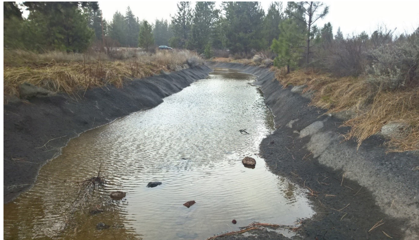
Concrete over geomembrane liner in test section A-2.
