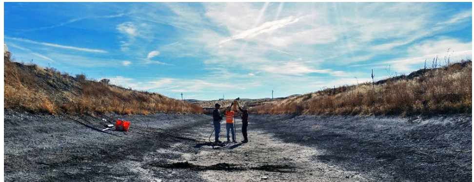
Installing field equipment in the Truckee Canal outside of Reno, Nevada.
