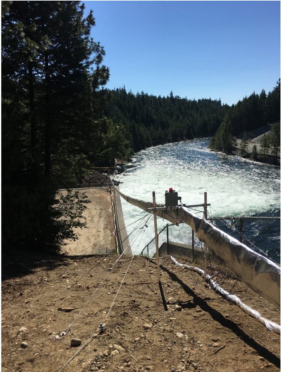
Whooshh™ transport tube next to Cle Elum Dam spillway, Cle Elum, Washington. Tube passed fish over the dam (1100' long and 165' high) just under an average of 60 seconds.
