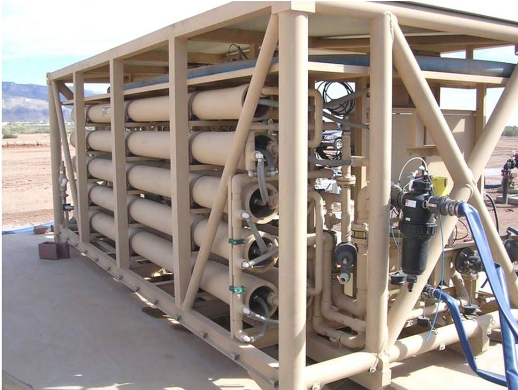
Figure 5-6. – RO skid showing RO vessels.
