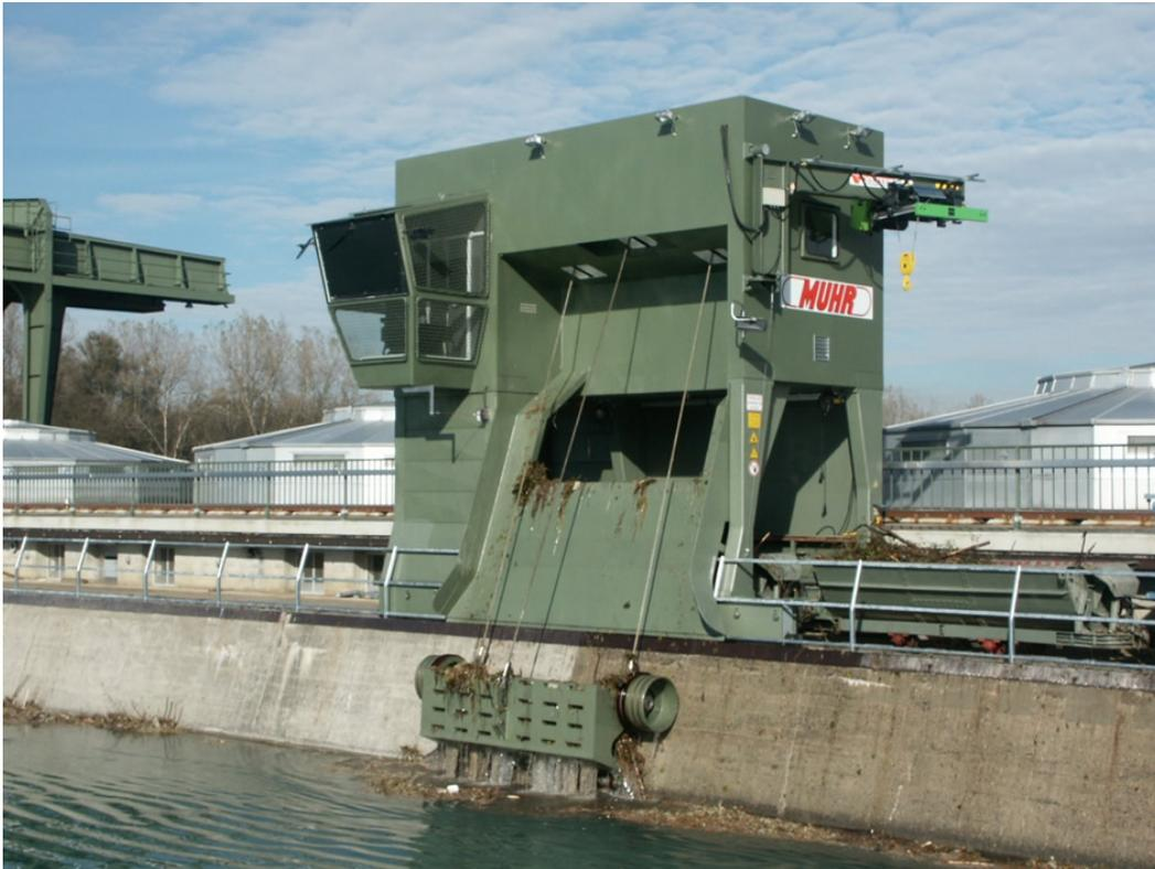
Figure 4 - Cable style rake on rails (image courtesy of lakeside-equipment.com)
