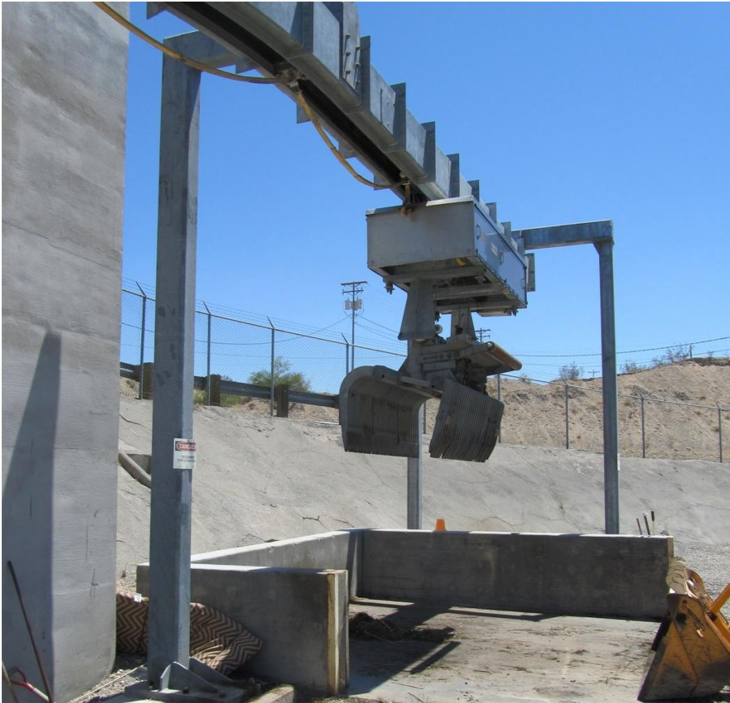
Figure 3 - Cable Style Rake and Gripper Head on Overhead Monorail on the Central Arizona Project.
