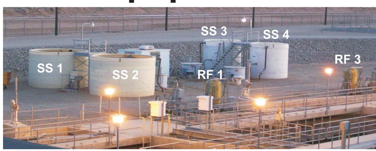
Figure 5. Slowsand pilot process area at the WQIC.
