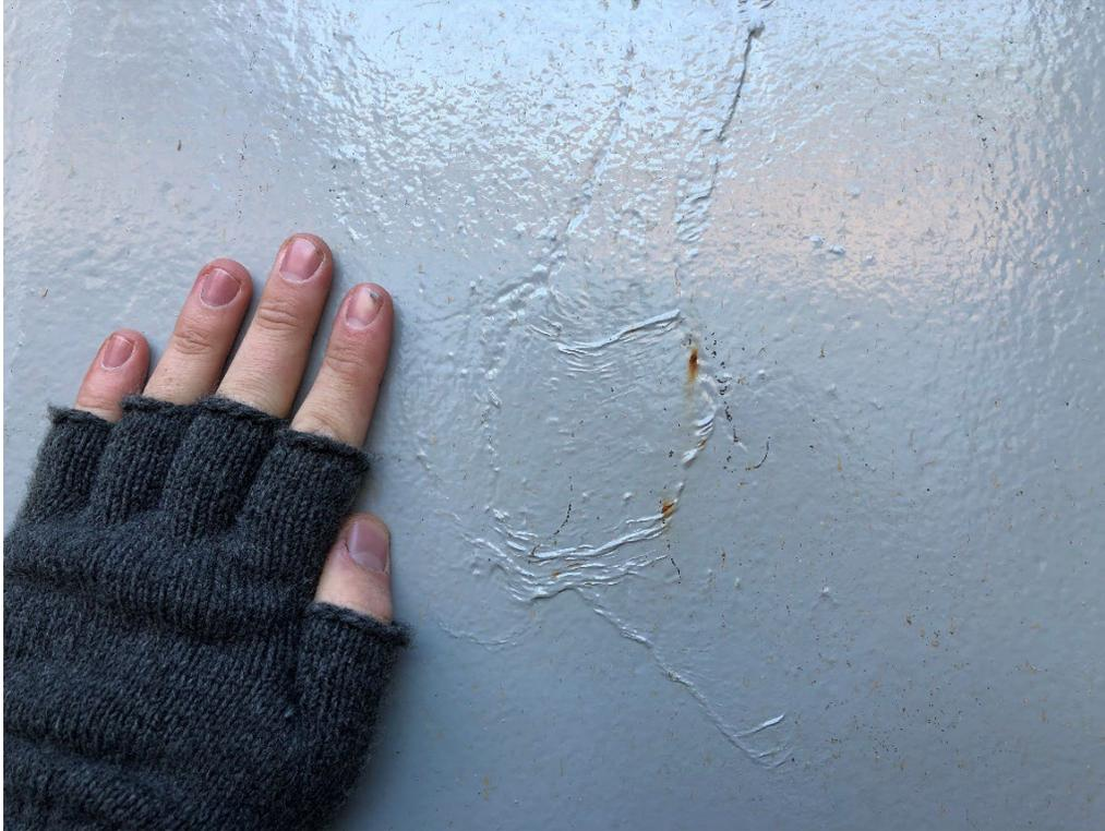
Figure 33: Sag of coating cause by excess buildup of coating during application. Cracking and corrosion have occurred.
