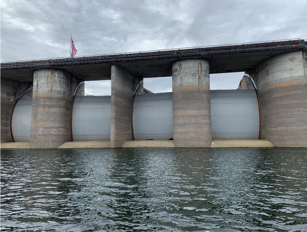
Figure 31: Upstream side of the four radial gates at Fontana Dam.
