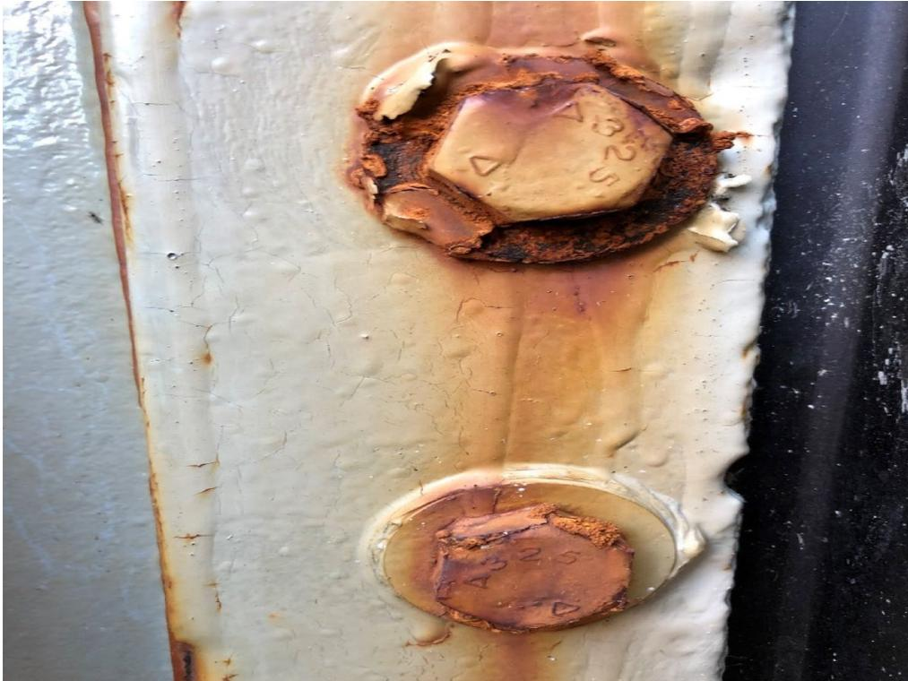
Figure 34: Micro cracking in coating, caused by excess film build up, on seal-clamp bars. Coating on bolts has become damaged and corrosion is present
