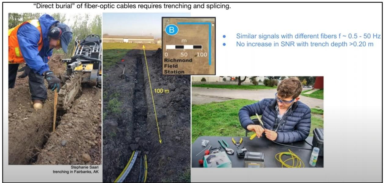
Figure 3 – Photographs showing the installation and splicing of DAS fibers at a site near Fairbanks, Alaska. Modified from Dou et al., (2017).
