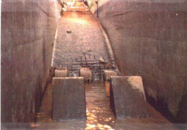
Figure 4. — Inspection photo from Taylor Draw Dam outlet works stilling basin, 1987.
