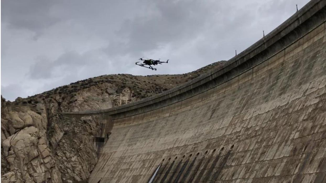
**Figure 33.—Intel’s Falcon 8+ UAS collecting inspection data at Arrowrock Dam, Idaho.**
