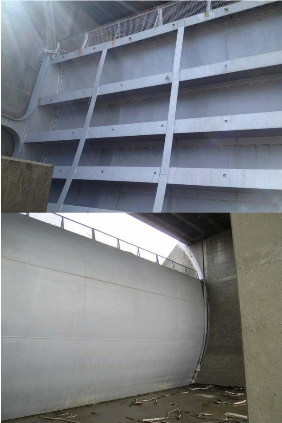
Figure 1. A radial gate at Cle Elum repainted in 1983 with Vinyl Resin VR-6
