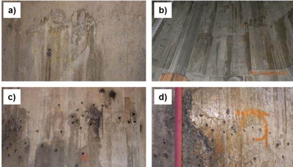
**Figure 14. Significant water flow from the cracks is shown in a) and b). The large number of grout ports is shown in both c) and d). The photo in d) also shows concrete spalling due to excessive pressure during grout injection.**
