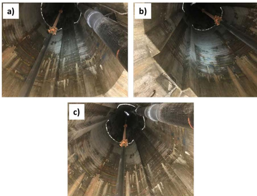
Figure 54. Photos were taken looking up from the bottom of the shaft. The photos in a), b), and c) all show new calcite formation over the first 12 months.
