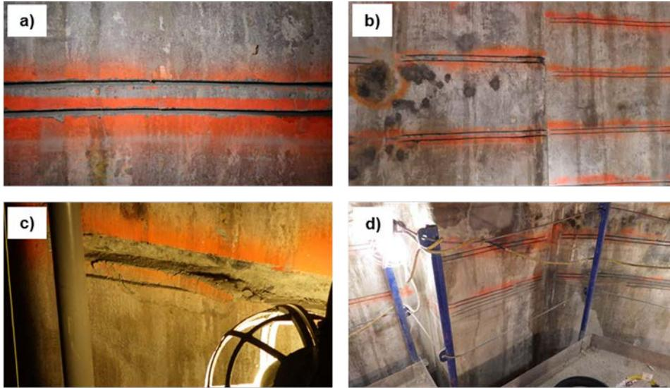
Figure 20. Anode grooves cut into the concrete wall. Photos a), b), and c) show cuts made prior to chipping out the concrete. Photos c) and d) show some chipped concrete and the results of extra cuts due to errors from the marks or labor.
