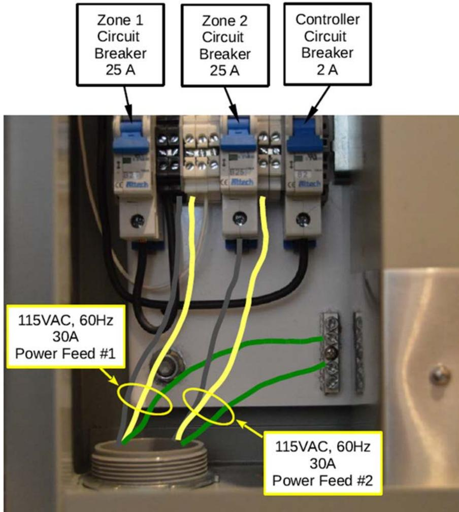
Figure 31. Input power wiring diagram.
