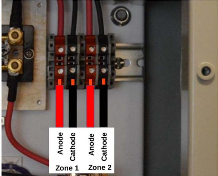
**Figure 34. Anode and cathode wire connections inside controller.**
