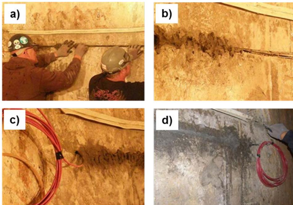
Figure 9. Installation of upper strip anode and hand packing of Portland cement grout into the groove shown in photos a), b) and c). Photo d) shows finished installation of upper anode strips and cable.
