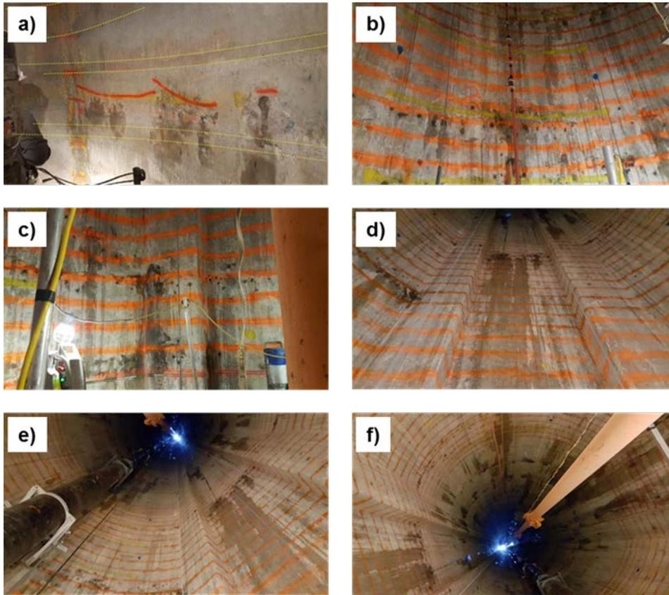
**Figure 19. Photos of shaft after marking the walls with paint indicating the location of the anodes. The photos show that some cracks were still leaking however most had been sealed.**
