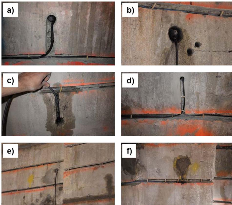
**Figure 25. Cathodes installed in holes drilled into the wall of the shaft. Note the cable is run back to the junction box in the same groove as the anode ribbons. The cathode and sensor probe holes were then packed with mortar as seen in f).**
