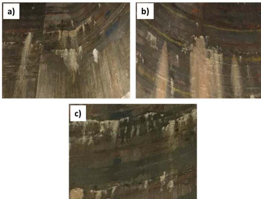
Figure 55. Photos were taken of the shaft in various areas in the EOP installation zone. The photos in a), b), and c) all show new calcite formation over the first 12 months.
