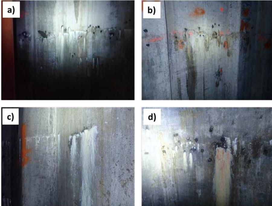
**Figure 51. Photos of areas above the EOP installation zones. Photos show locations where grouting was performed which are still leaking and areas of cracks which were not grouted.**
