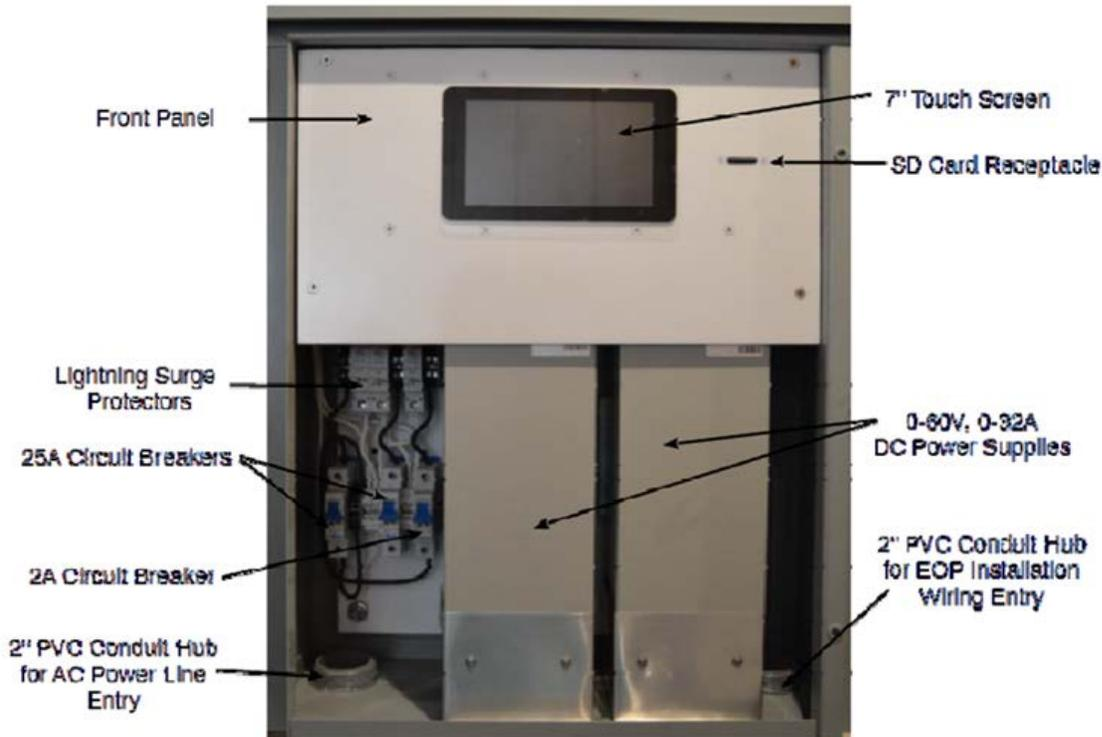
**Figure 29. EOP controller for operating the system by applying a pulse sequence to the installation.**
