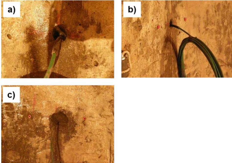
**Figure 10. Installation of strip cathodes into holes drill to a depth of ~18 inches shown in a) and b). Portland cement grout was poured in the holes around the cathodes, and the cathodes and cables were grouted in as shown in c).**
