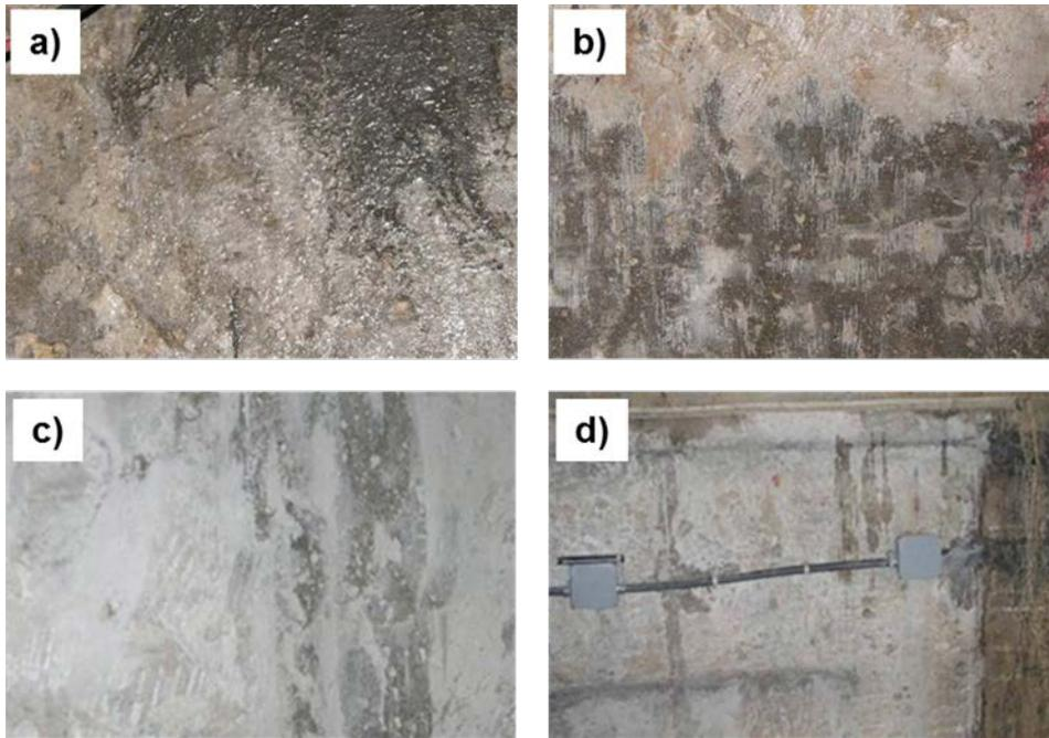
**Figure 12. Condition of wall at installation prior to energizing of the system is shown in a) and b). Note the wall was damp to sight and touch. The wall was dry to sight and touch over most of the test section after two weeks of system operation as shown in c**
