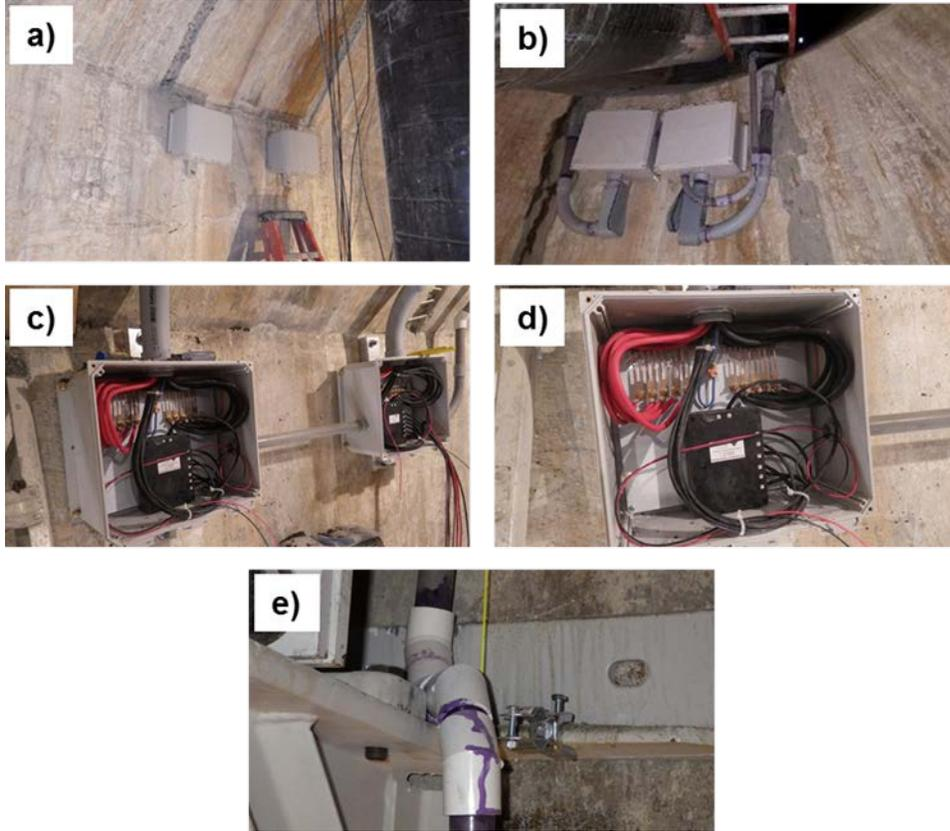
Figure 28. Junction boxes mounted at the top of the bonnet cover chamber, a) and b). Photos c) and d) show the cable connections inside the junction boxes, including cathode and anode cables. Photo e) is the conduit for the cables connecting to the EOP controller.
