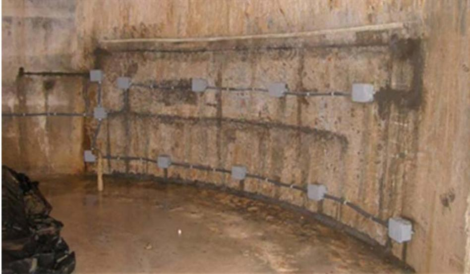
**Figure 11. Completed installation with junction boxes and conduit.**
