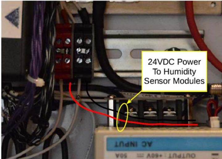
**Figure 35. 24 VDC humidity sensor interface power connections.**
