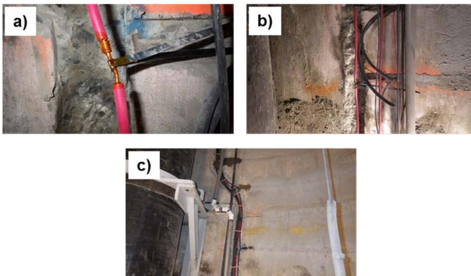
**Figure 23. Anode ribbons crimped to a copper cable is shown in a). Photos b) and c) show the cables placed in a groove cut into the wall and running to the junction box.**
