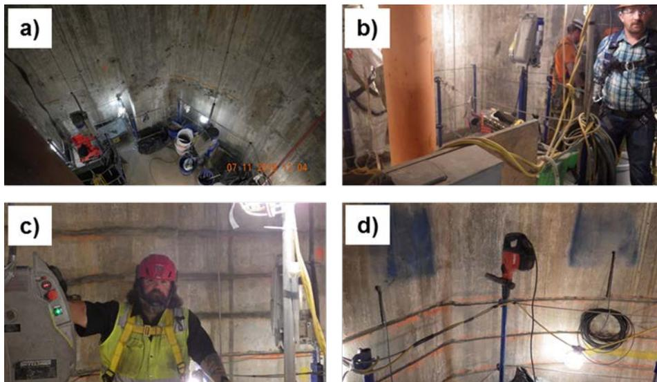
**Figure 18. Installation was performed using a traveling platform.**
