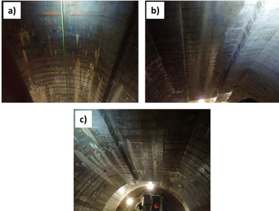
Figure 53. Photos were taken looking down the shaft from above. The photos in a), b), and c) all show new calcite formation over the first 12 months.
