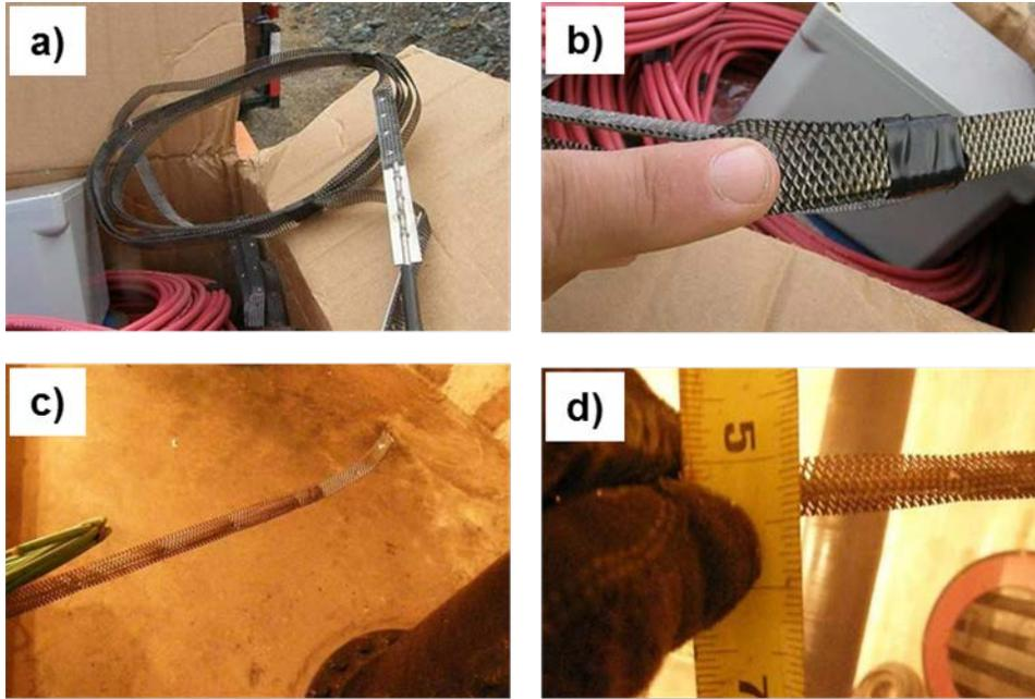
Figure 8. Mixed metal oxide coated titanium mesh strip type anodes (a and b) and cathodes (c and d) installed in the concrete wall.
