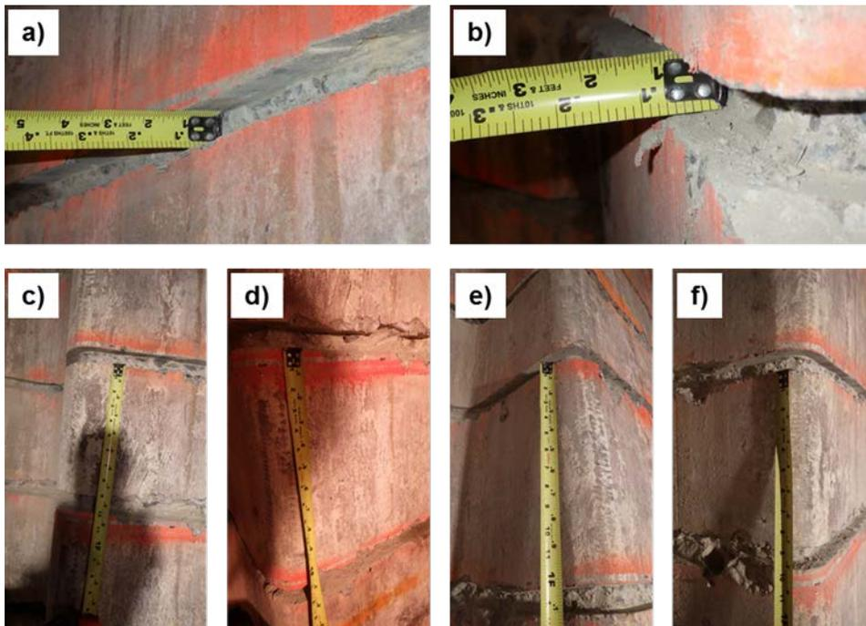
Figure 21. Dimensions of a representative number of anode grooves cut into the walls. These photos indicate that the grooves and therefore the anodes were not always separated by a foot.
