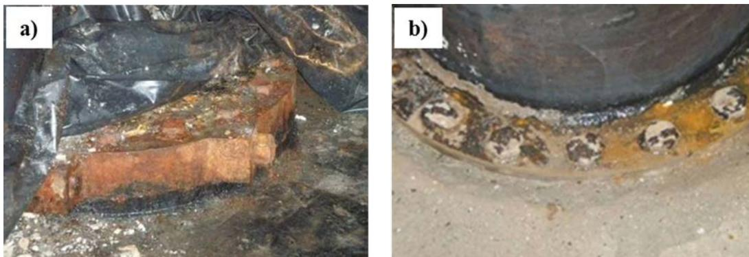
Figure 1. Corrosion of the bonnet cover and air inlet pipe due to the standing water.
