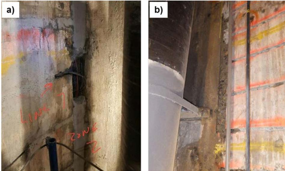
**Figure 27. Cable trench for terminating anode ribbons, cathode cables, and sensor probe cables from each section. Trenches were packed with mortar to embed the cables.**
