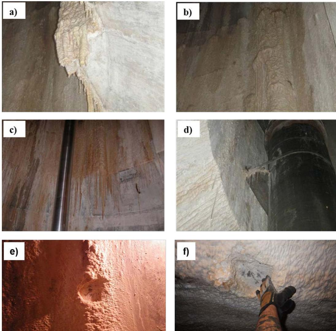
**Figure 2. Calcite deposits observed on the walls of the headgate shaft. Excessive seepage over time has resulted in stalactites and corrosion of air vent supports.**
