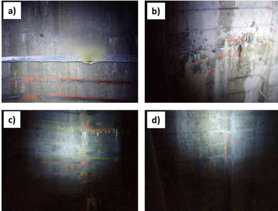
**Figure 52. Photos from the EOP zone indicating water coming from above and from cracks in the EOP zone. The photo in a) shows the calcite building up on the drip tray which was installed. The photos in b), c), and d) shows calcite build up due to seepage from cracks which were not successfully grouted.**
