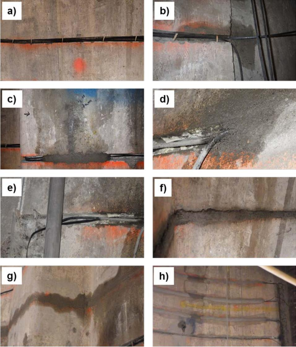
Figure 26. Photos showing cables from cathodes and sensor probes in same grooves as anode ribbons. Grooves were then packed with mortar.
