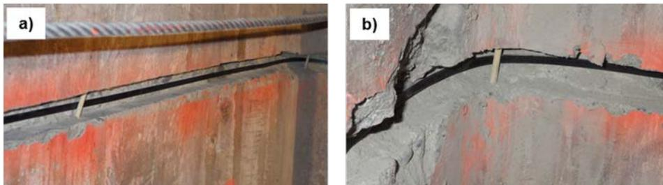
**Figure 22. MMO anode ribbons installed in grooves and held in place using wooden dowels.**
