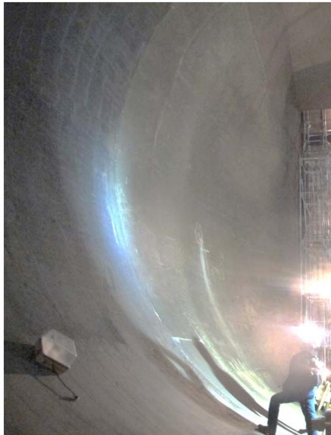
**Figure 1: Hand-applied coal tar enamel with minimal damage after 40 years in large penstock.**
