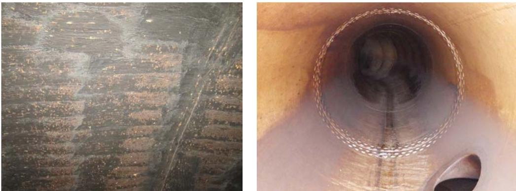
**Figure 2.—Penstock interiors lined with (left) original coal tar enamel at Grand Coulee Third Powerplant and (right) new polyurethane after several years of service at Flatiron Powerplant.**
