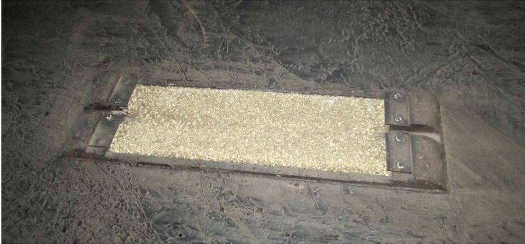
**Figure 3.—Sacrificial anode for GACP system within penstock at Grand Coulee Third Powerplant.**
