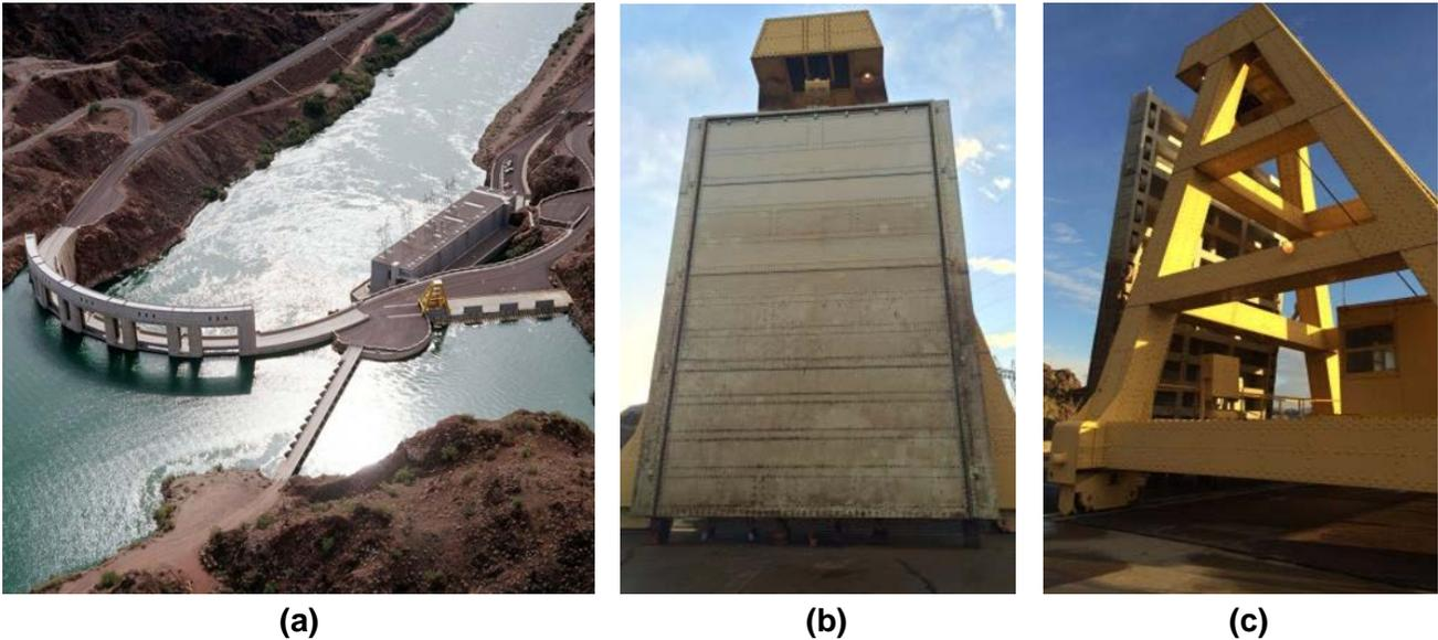
**Figure 2: Parker Dam (a) has four penstock gates on the west (right) side of the main river; a hoist crane is used to access the (b) upstream and (c) downstream sides of the penstock gates.**
