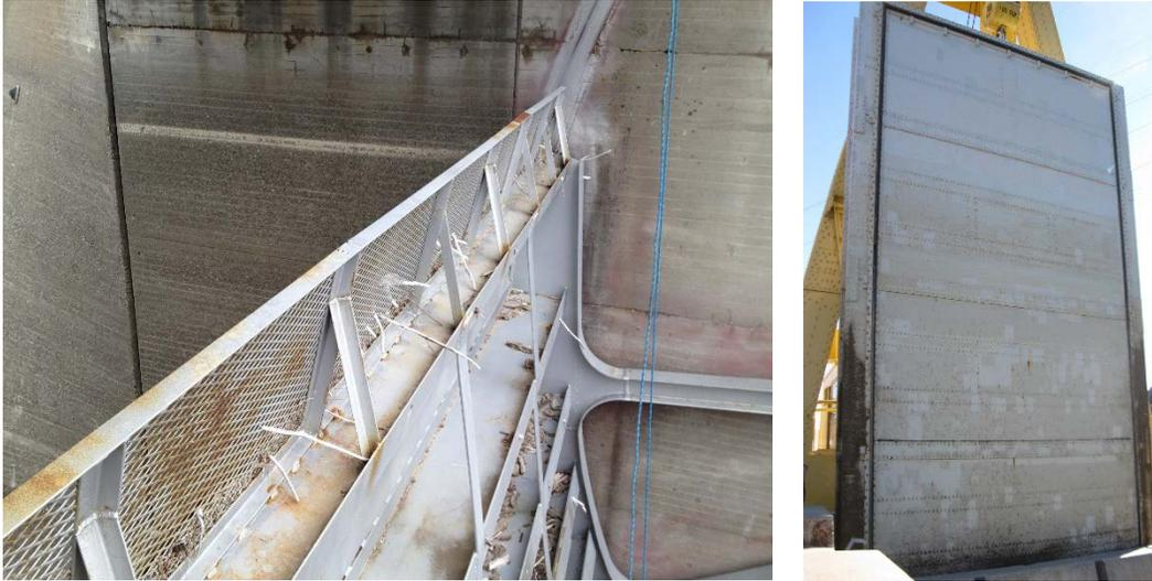
**Figure 4.—(left) Radial gate at Cle Elum Dam with vinyl paint exposed to woody debris and (right) bulkhead gate at Parker Dam with epoxy coating that has received spot repairs.**
