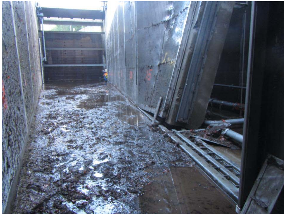
Figure 9. Screen damage on a flat plate screen from excess head pressure (Soda Springs Dam fish screen, Umpqua, OR).
