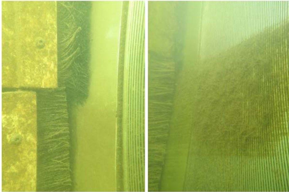
Figure 13. Brush misalignment from a NMFS dive inspection showing a section of fish screen that is not being cleaned properly (Natomas Mutual Water Company, Sankey water intake and fish screen, Natomas, CA).
