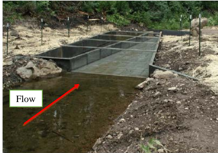
Figure 4. Horizontal flat plate screen diversion (East Fork Ditch Company, ID).
