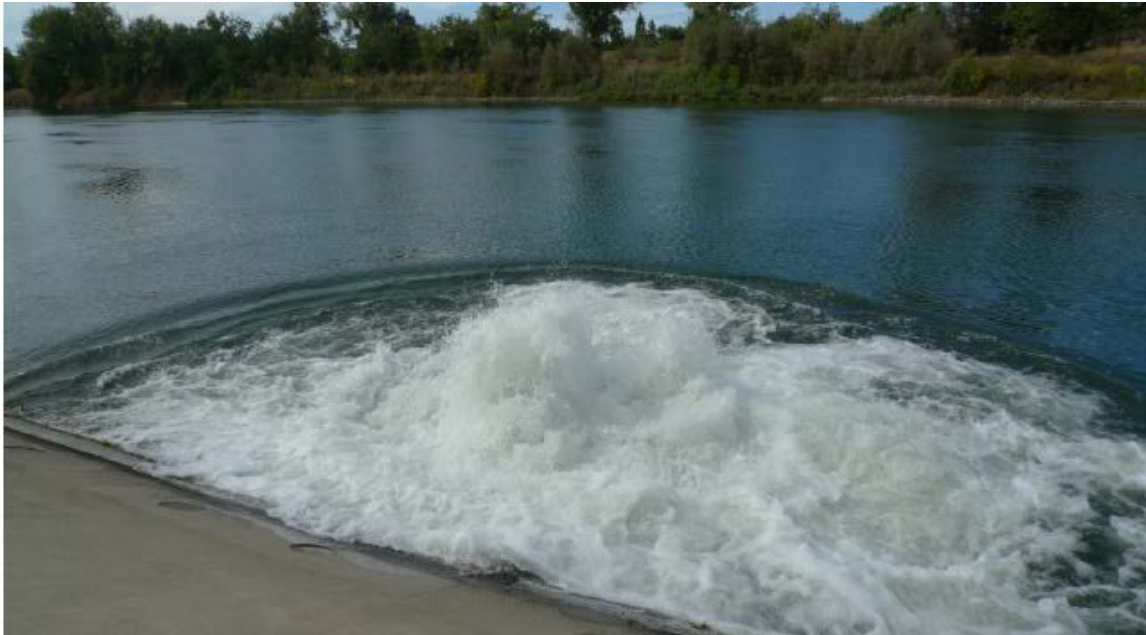
Figure 11. Air burst cleaning at Reclamation's Princeton Pumping Plant (Princeton, CA).
