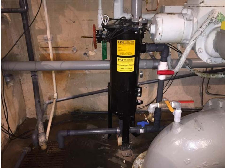
Figure 5. Bag filter housing installed on purge line to collect debris removed by separator
