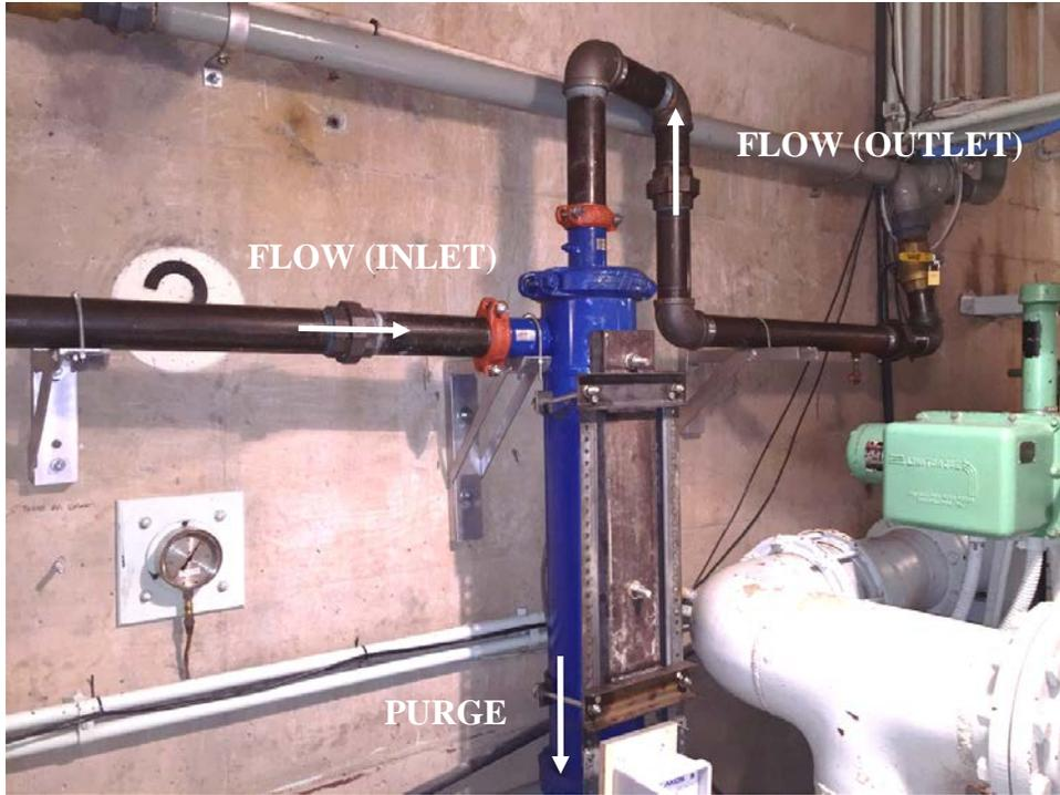
Figure 4. Centrifugal separator installed on test branch
