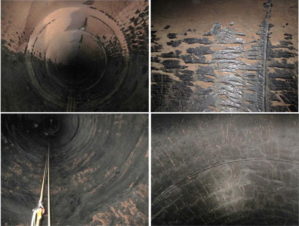
**Figure 22. Coal tar enamel hand-dauber degrees of degradation in service: (top-left) severe with close-up at (top-right), (bottom-left) moderate, and (bottom-right) minor-to-moderate.**
