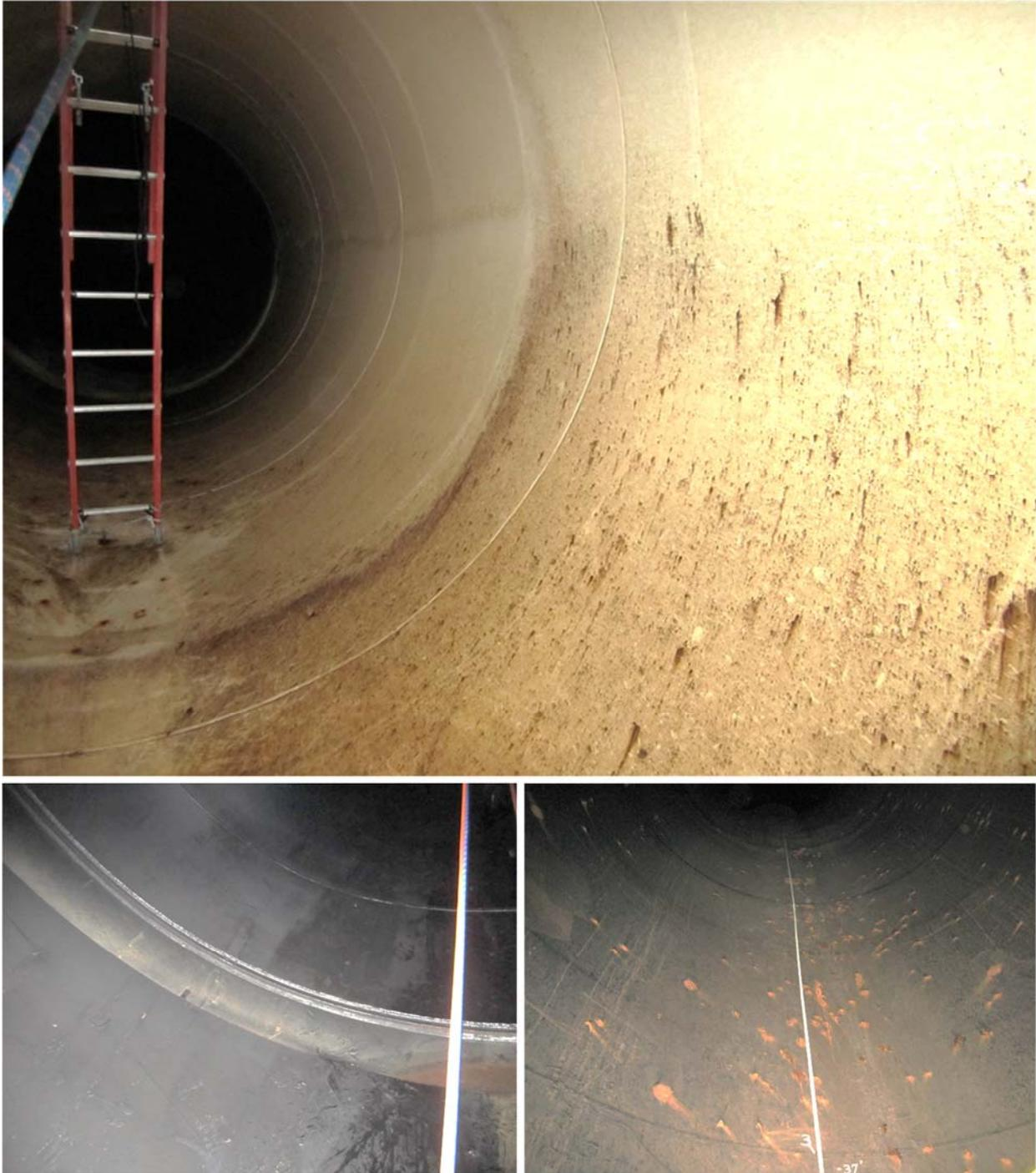
**Figure 23. (top) Assumed to be epoxy coating with moderate degradation and coal tar epoxy (bottom-left) in good condition and (bottom-right) with moderate degradation.**
