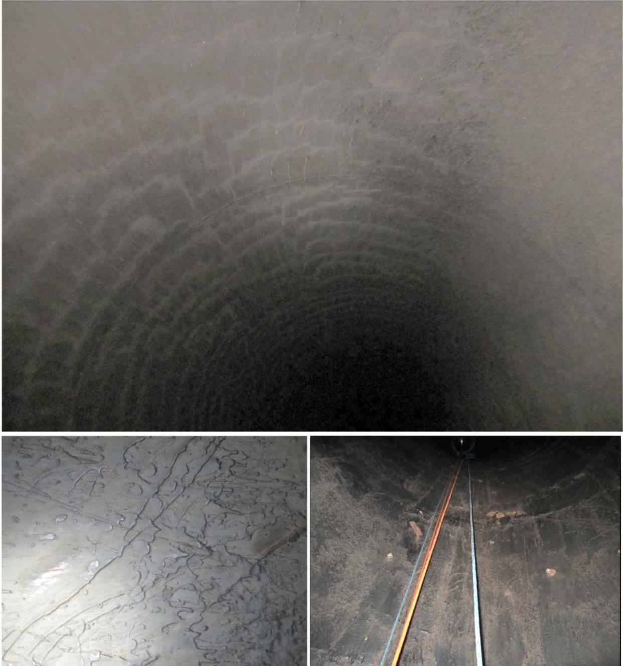
**Figure 21. Coal tar enamel (top) applied by hand-dauber in good condition, (bottom-left) applied by mop in good condition, and (bottom-right) applied by hand dauber beginning to crack, chip, and degrade.**
