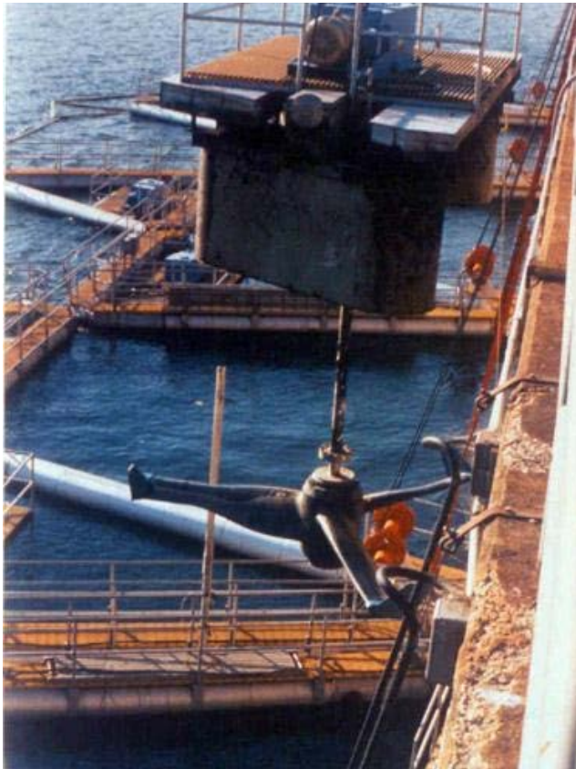
Figure 2. Large surface water pump being installed (credit to Mobley Engineering, Inc.)
