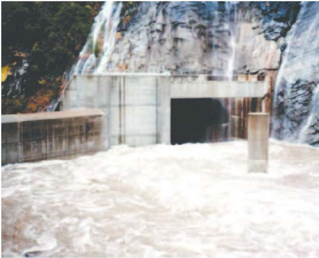
**Figure 6: Pile upstream of tunnel entrance, intended to rotate debris to pass through the tunnel (Photo credit: Eberhardt et al., 2007).**
