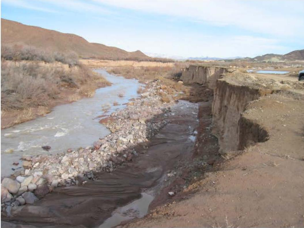
**Figure 1. Location of Homestead Weir prior to weir construction and restoration, showing evidence of significant downcutting and erosion.**
