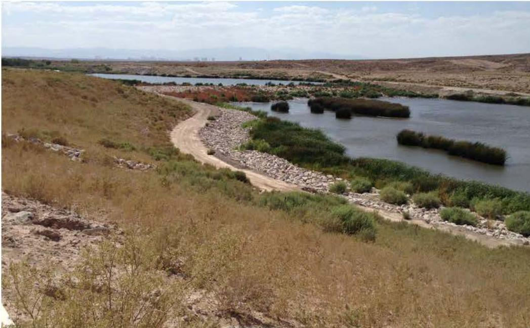
**Figure 2. Homestead Weir in 2014. The weir was completed in 2011 and is constructed from rock rip rap, allowing water to flow through the structure. Riparian vegetation planted on the weir and along the banks of the Wash upstream also contributes to channel stabilization.**
