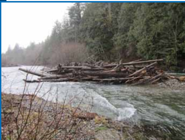
A multilog large wood structure placed in the center of the Green River, a tributary of the Colorado River.
