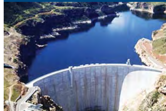
Yellowtail Dam, Montana.
