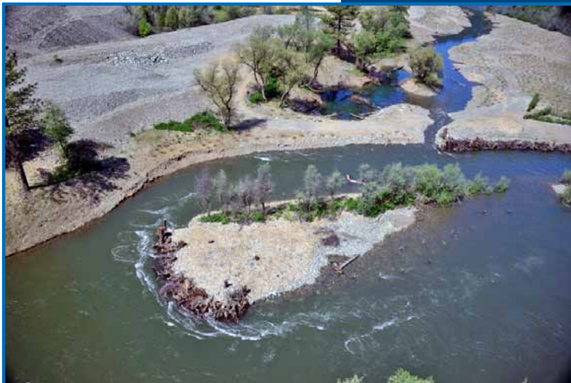
Engineered logjam on the Trinity River under floodflows. Photograph courtesy of the Trinity River Restoration Program.
