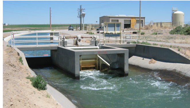
Check structure on the Amarillo Canal, Farmington, New Mexico
