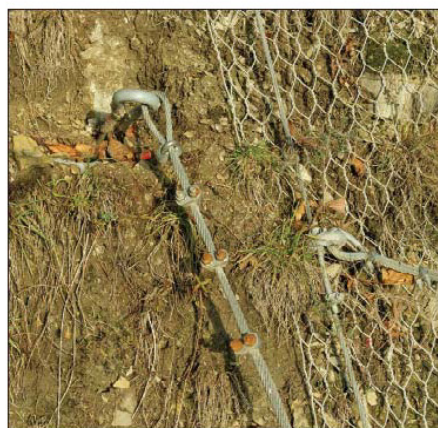
Rotary UAS can be used to assess the precise condition of rockfall protection netting.
