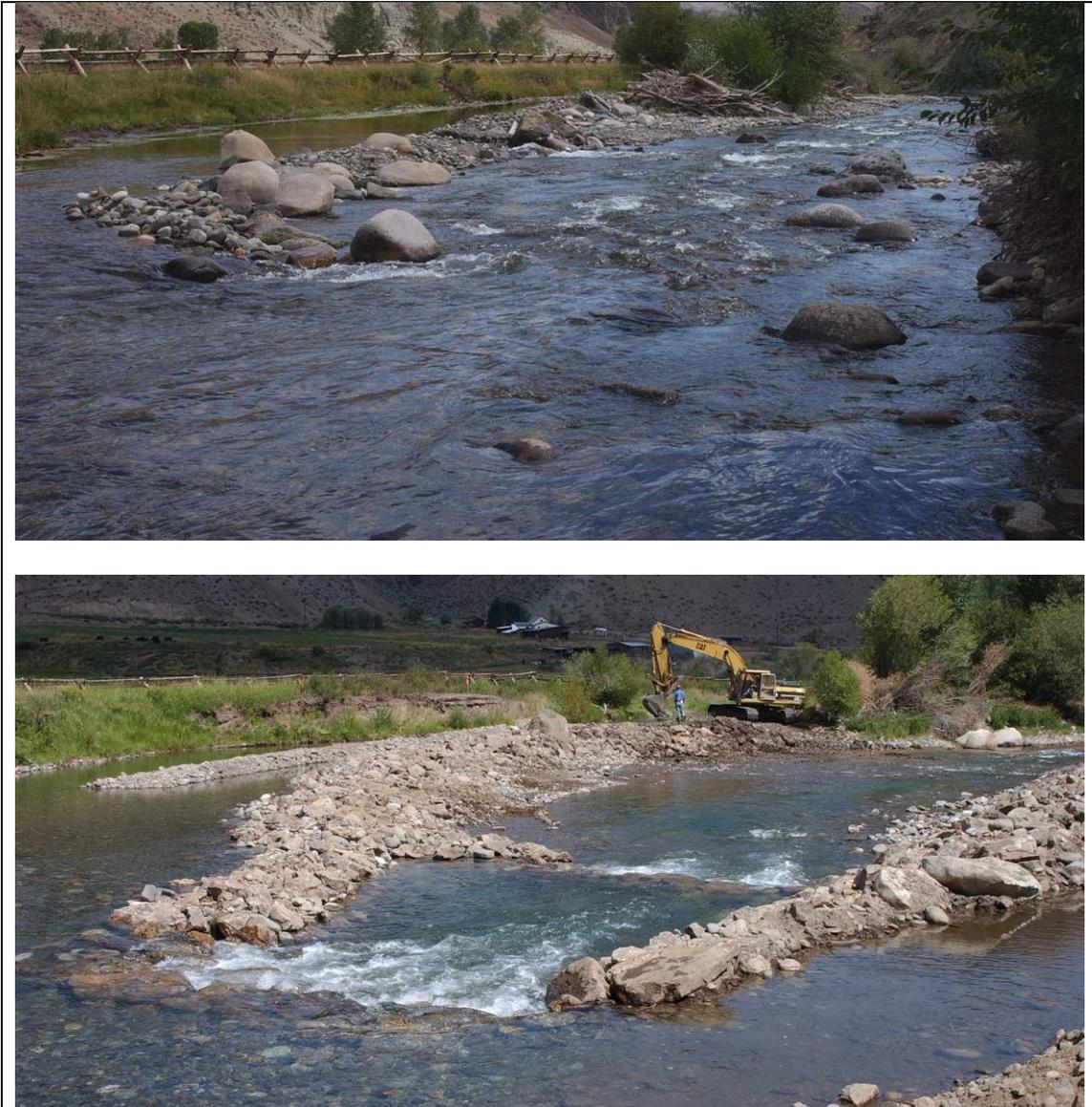
**Figure 21. Pre- and Post- construction photos on the East Salmon River. Note changes in velocities and water surface profiles. East Fork Salmon River, ID**
