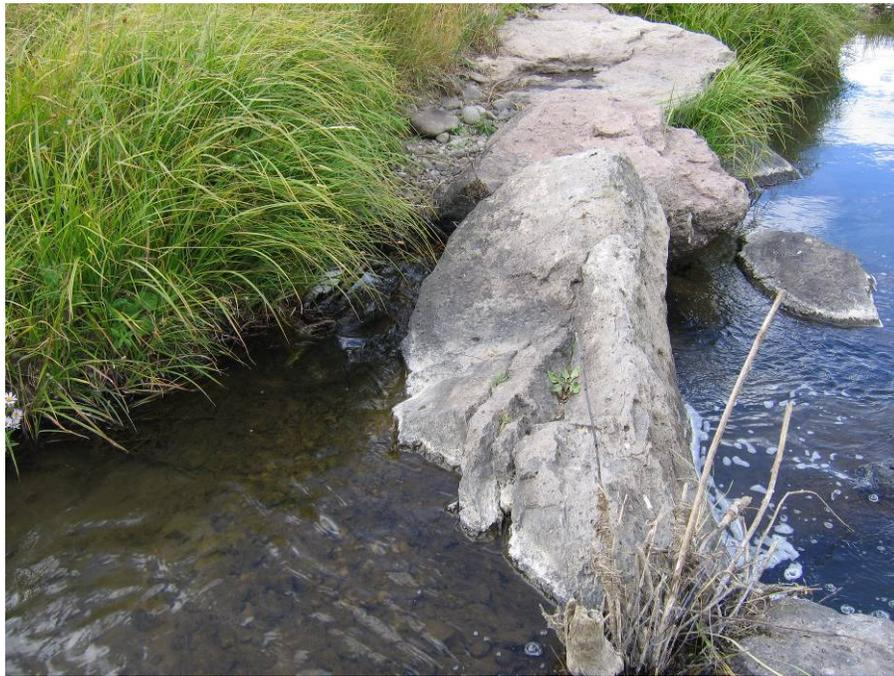
**Figure 22. Footer pushed out, header tilted upstream. Little Snake River, CO.**
