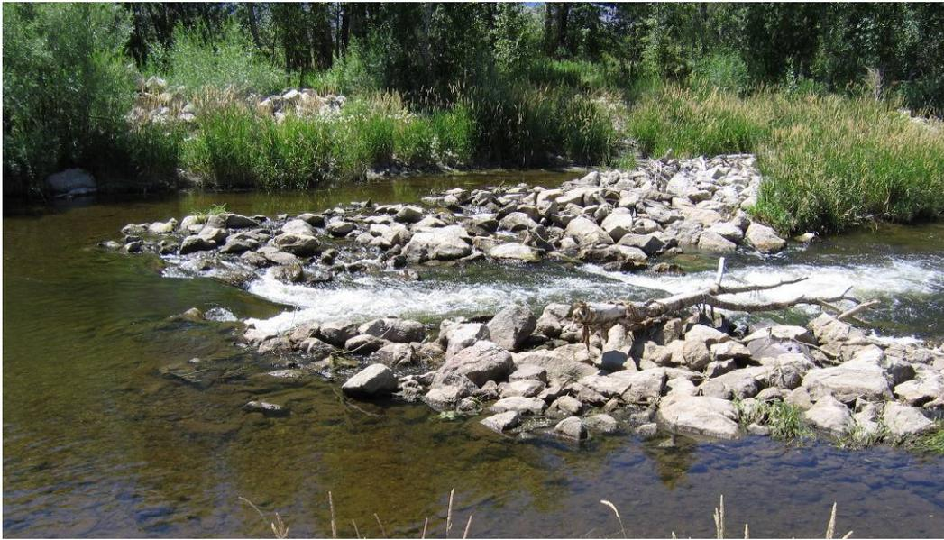
**Figure 19. Steep sloped ramps frequently used in PN Regional Designs. Lemhi River, ID**
