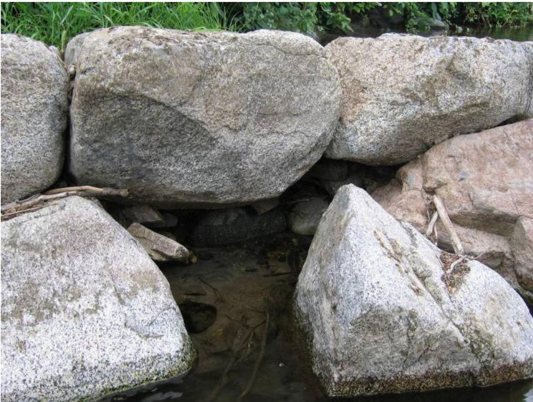
**Figure 28. Interlocking of rocks providing additional structure support.**
