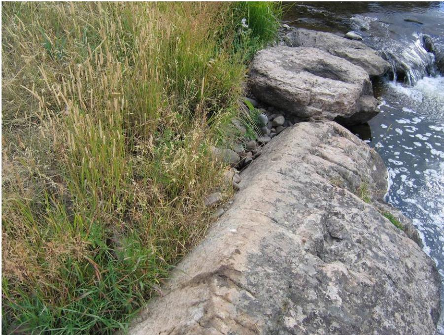
**Figure 24. Header/footer pulled away from bank. Little Snake River, CO.**
