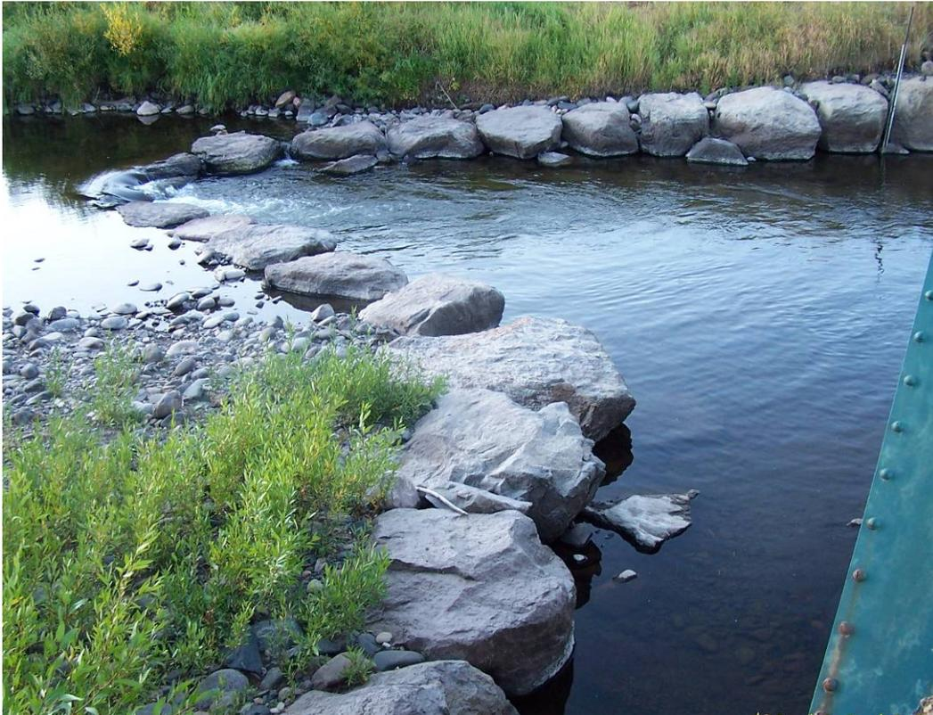
**Figure 20. Typical Rosgen design with a single rock width of rocks defining structure. Little Snake River, CO**
