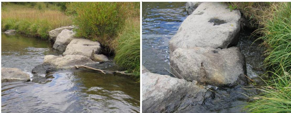
**Figure 27. Piping through the Arm Resulting in Flanking. Little Snake River, CO.**
