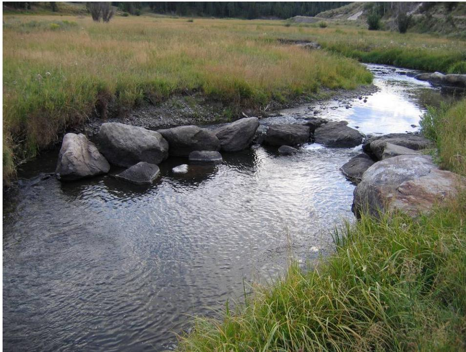
**Figure 7. Structure without a tie-in showing flanking around the right arm. Little Snake River, CO.**
