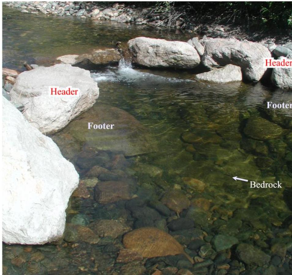
**Figure 11. Header-Footer configuration with exposed bedrock in scour pool. Little Snake River, CO.**
