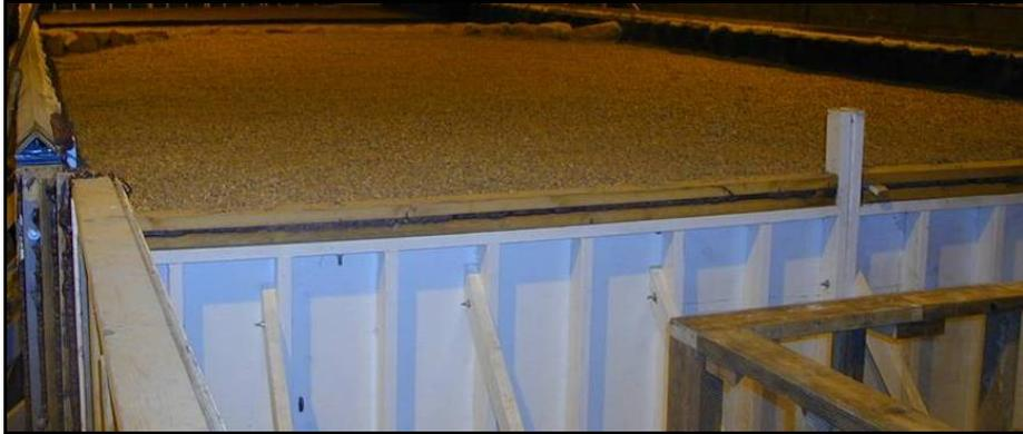
**Figure 2.5. Photograph of Stop Logs**
