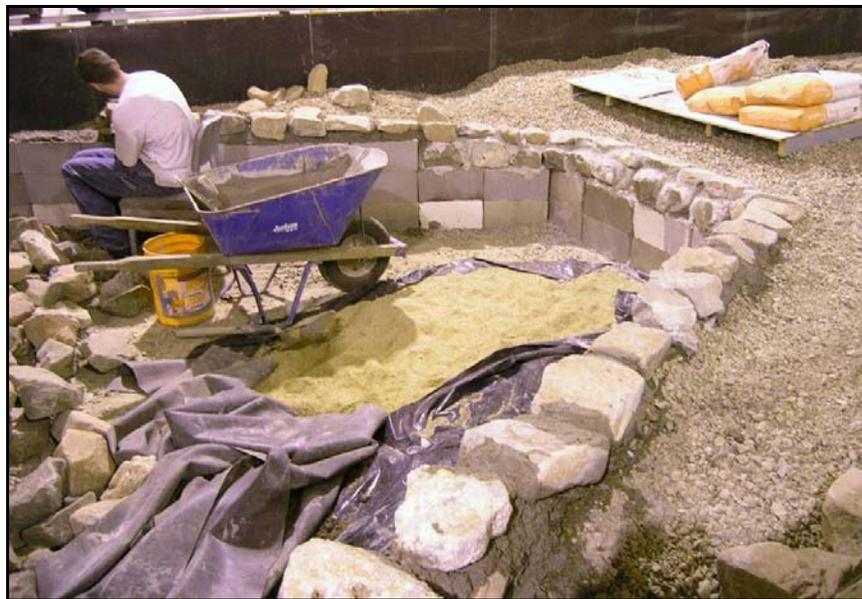
**Figure 3.2. Photograph of Anchor Wall and Grouted U-weir Construction**
